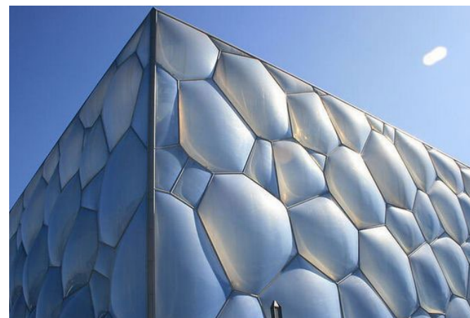
Figure 71 | ETFE pillow facade. Beijing National Aquatics Center by Arup, 2008. cross section. source: http://www.etfe-cushions.com/sell-translucent_etfe_cushion_facade_triple_layer_etfe_pillows_etfe-2117959.html
