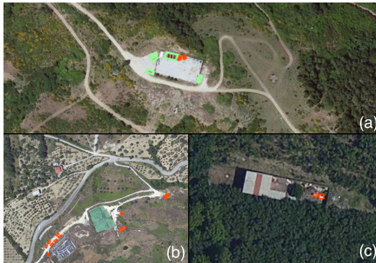
Figure 5.19: Example of atypical wastes in rural areas. In sub-image (a) it possible to see a group of dumpsters (in green) and a group of pallets (in red), in sub-image (b) there is a large group of dumpster (in red) found in an illegal landfill placed in a rural areas and in sub-image (c) it is possible to see two IBC (in red) with around scattered wastes in the middle of a wood. These annotations are opportunely made to provide insight only on these specific classes in rural areas and do not reflects annotation strategy used for the dataset.
