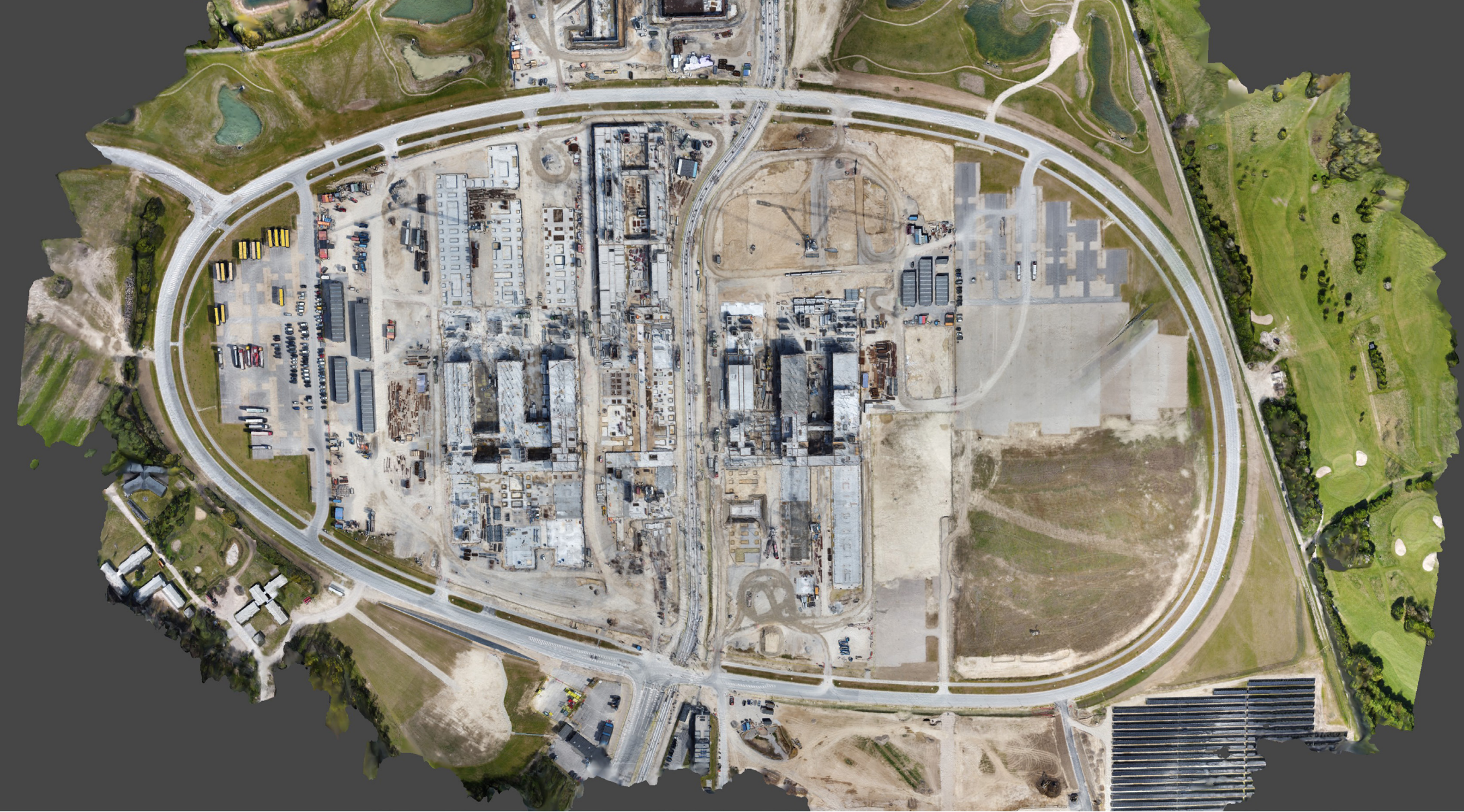
NYT OUH ongoing construction scanned by drone using pointcloud by author
