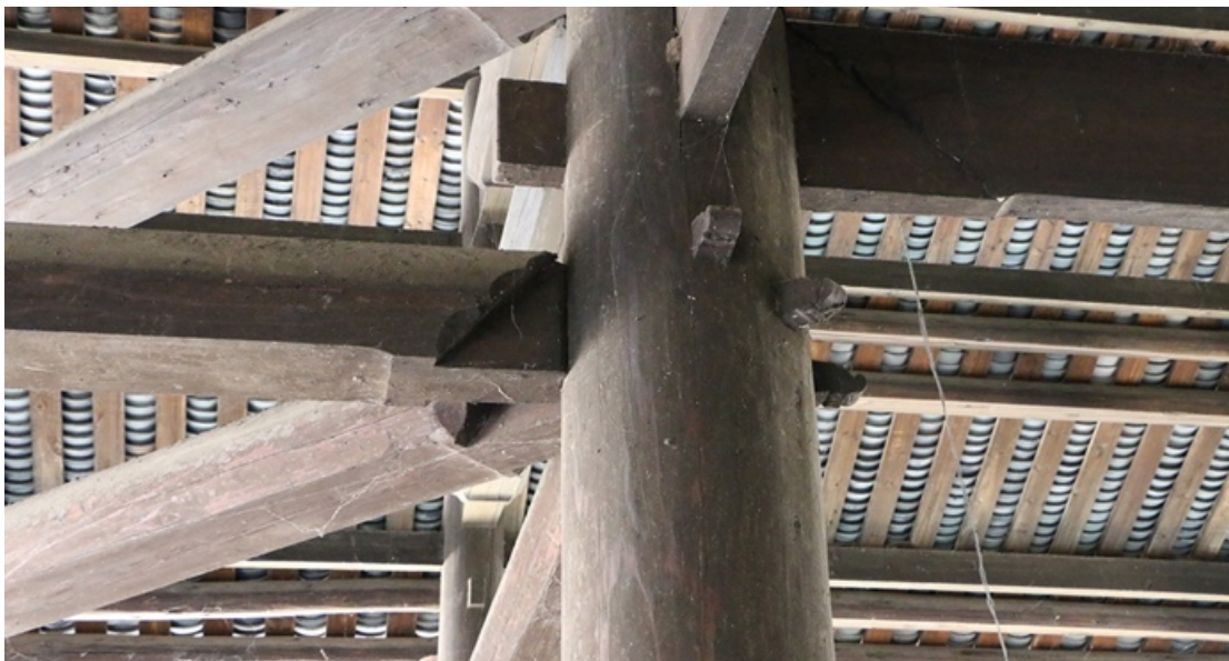
Fig.1-26 Tie beams arranged at different heights (Photograph by author, 2018)
