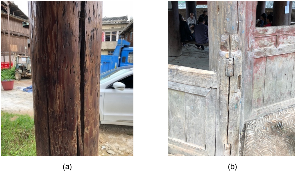
Fig.3-8 Splitting and checking on elements (Photograph by author, 2018)
