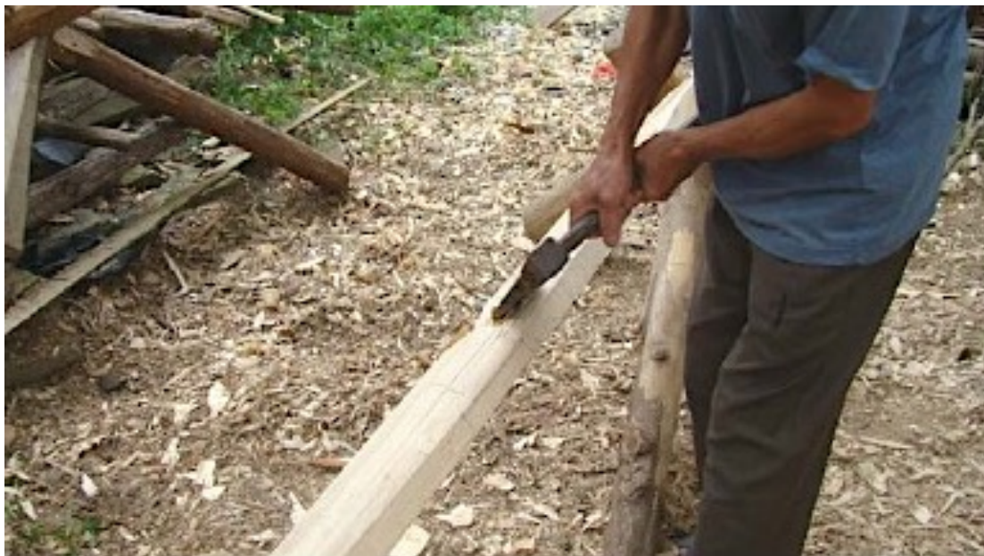
Fig.1-44 Axes for Dong carpenters (Photograph by author, 2018)
