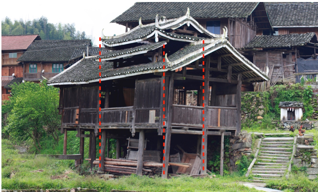
Fig.3-12 Overall tilt of Xiaozhai Drum Tower (Photograph by author, 2015)
