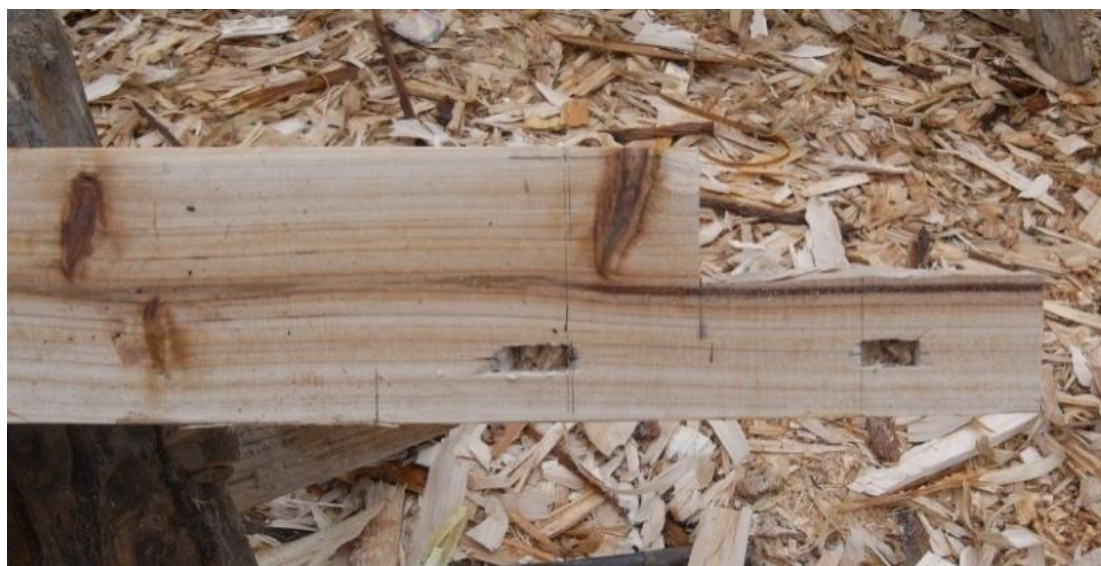
Fig.1-38 Knots in the processing of a tie-beam (Photograph by author, 2018)
