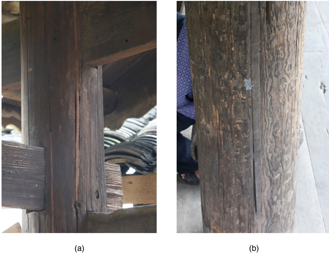
Fig.3-30 Wood patching method (Photograph by author, 2018)
