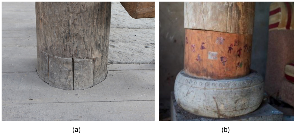
Fig.3-31 Splicing joint method in the foot of column (Photograph by author, 2018)
