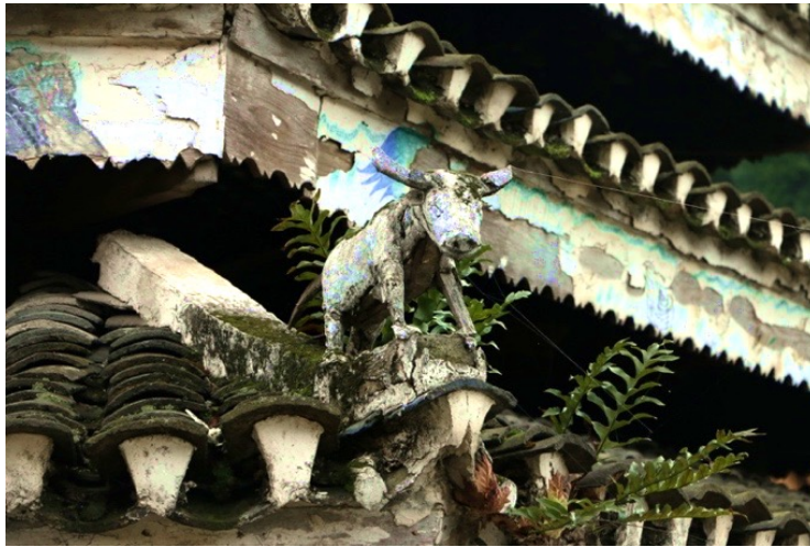
Fig.1-64 A buffalo sculpture on the roof corner (Photograph by author, 2018)
