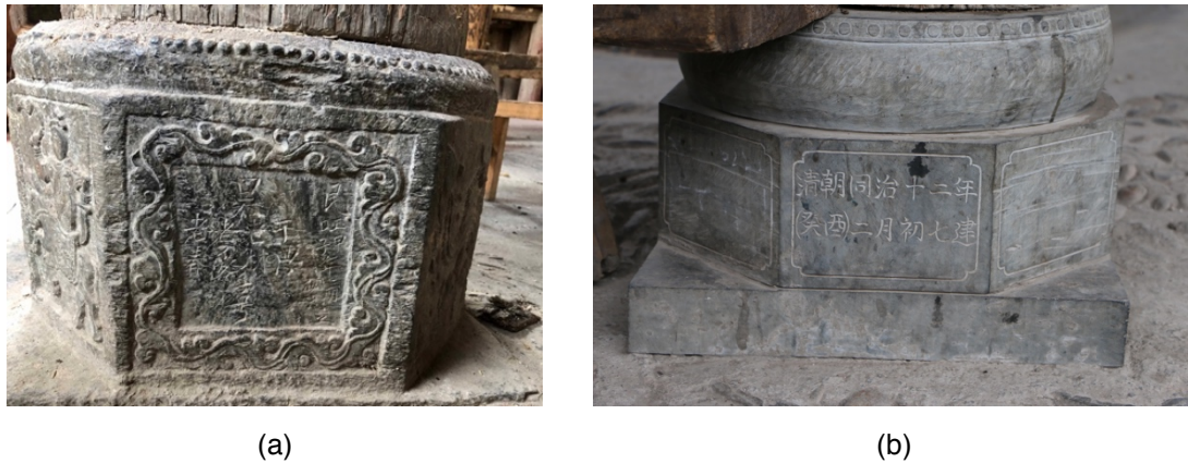
Fig.1-34 Column base with construction date in lunar calendar (Photograph by author, 2018)
