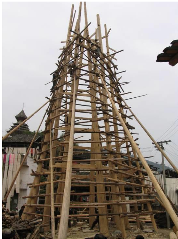
Fig.1-60 The procedure of frame erection (Photograph by Derong Kong, 2015)
