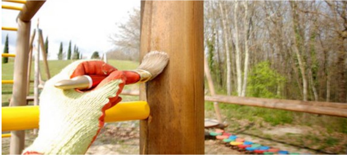
Fig.4-17 Brushing preservative on timbers
