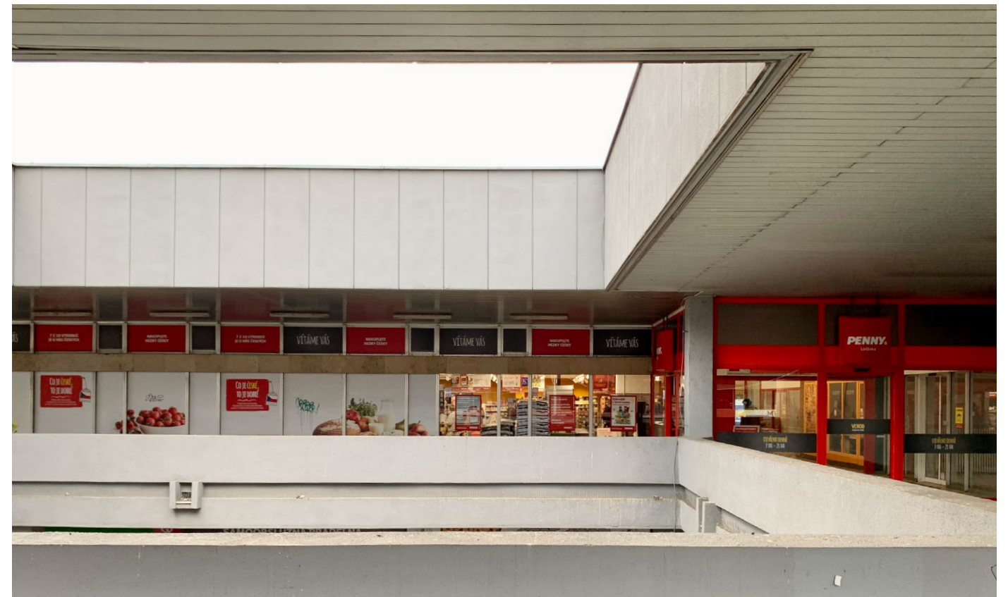
Fig. 29 Blocked portico in the first floor as the new entrance hall for the supermarket Penny. © Rudolf Nikerle
