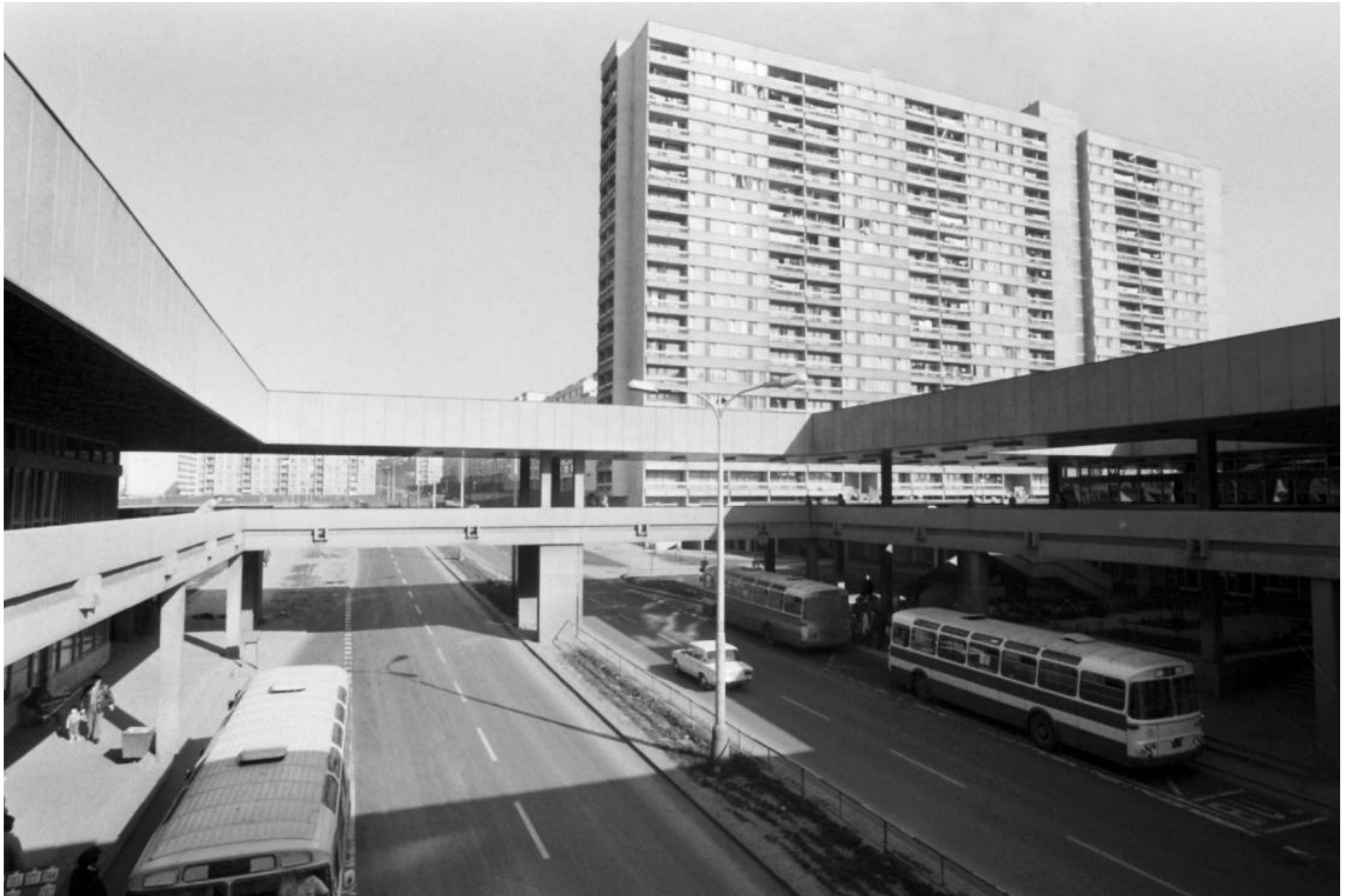
Fig. 8 Odra view from the bridge. © Odra 1.4.1980. Šourek Jiří, Humpálová Zuzana, Sýbek Jaroslav, ČTK
