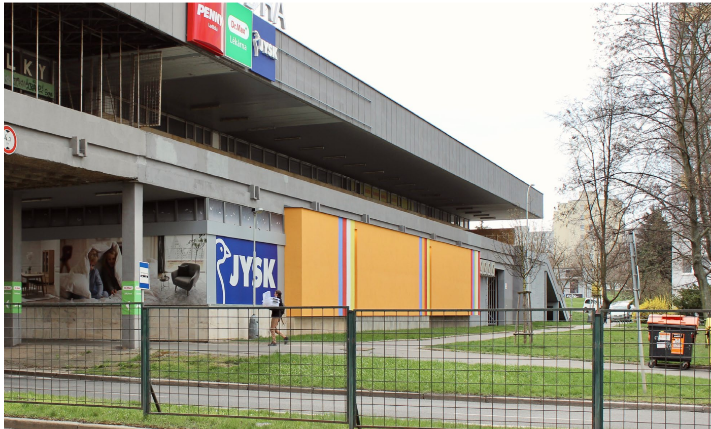
Fig. 26 West facade with visible expansion of JYSK shop replaced original portico. Missing outside staircase demolished in 2017. © Rudolf Nikerle
