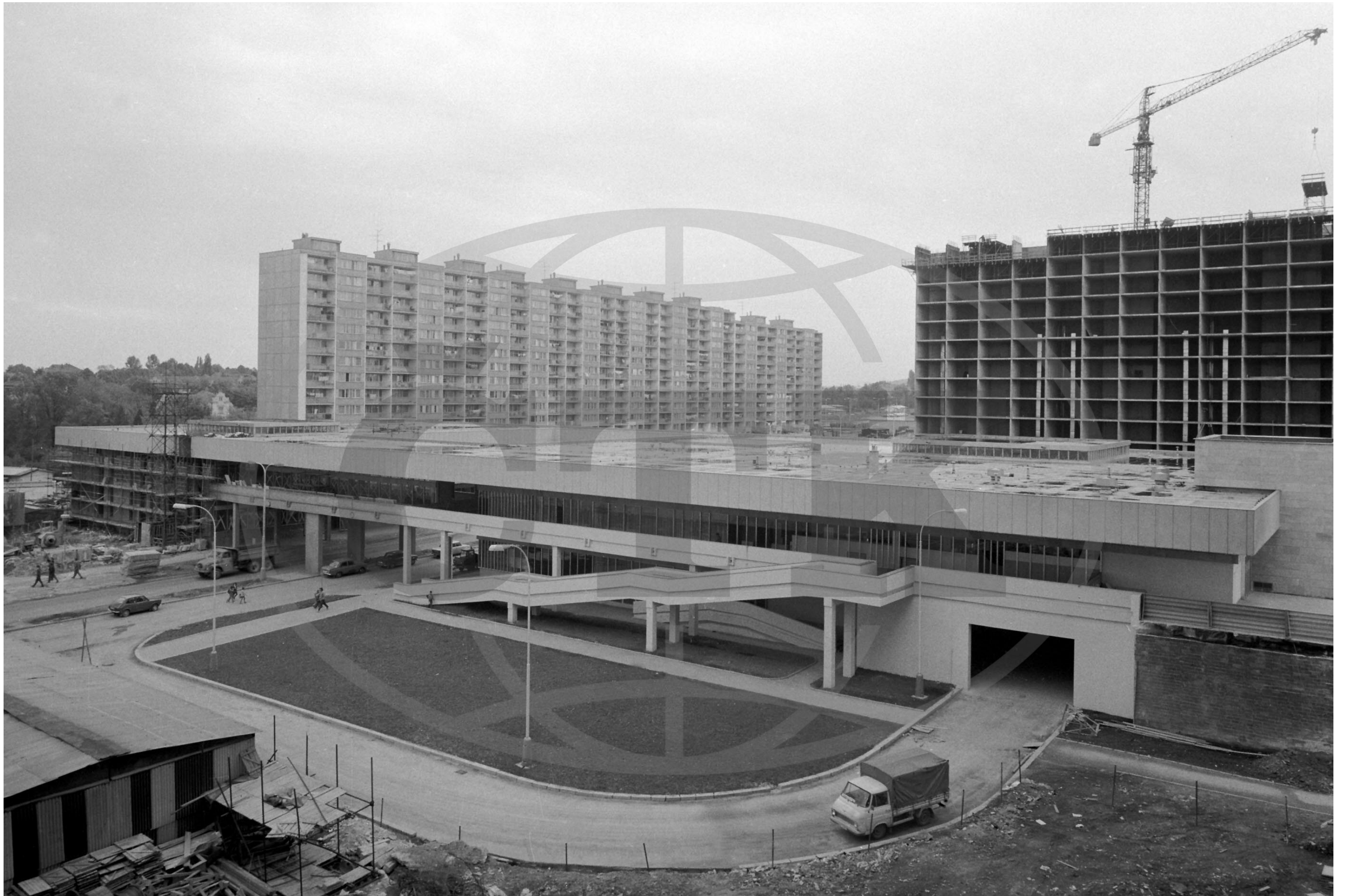
Fig. 24: Odra during construction works. © Odra 8.7.1976. Sýbek Jaroslav, ČTK
