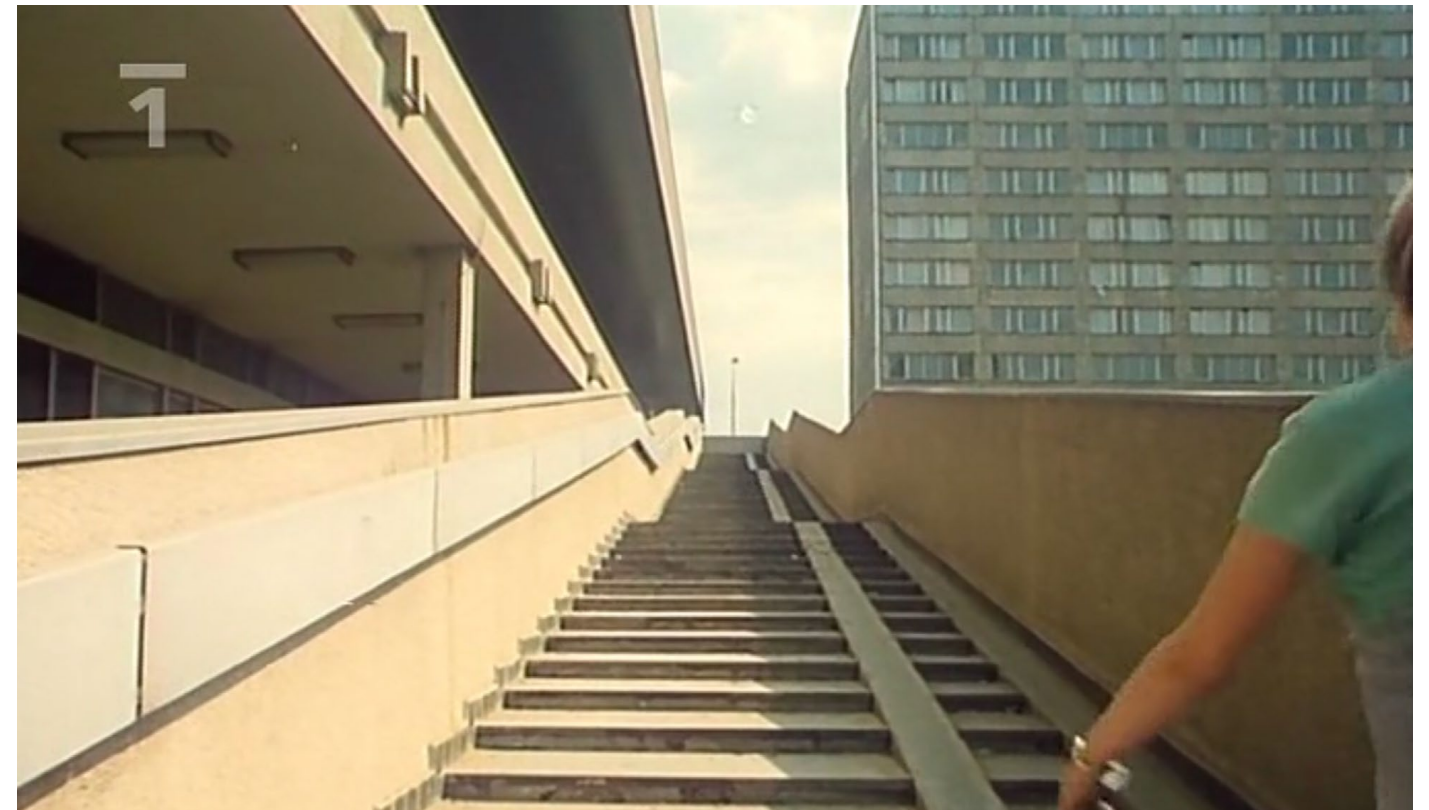
Fig. 18: Odra original exterior appearance of concrete staircase with concrete railings. © Čekání na déšť, 8.7.1978. Karel Kachyňa
