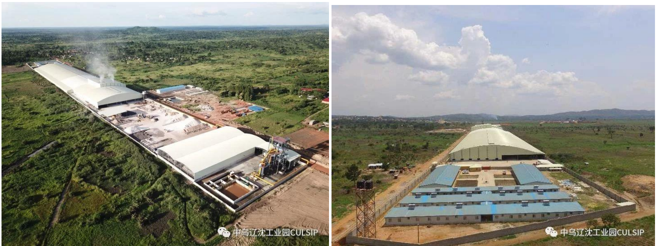
Figure 56: Pictures showing the factory building typology and layout in the Goodwill Uganda Ceramics Industry (Source; USLIP, 2018)
