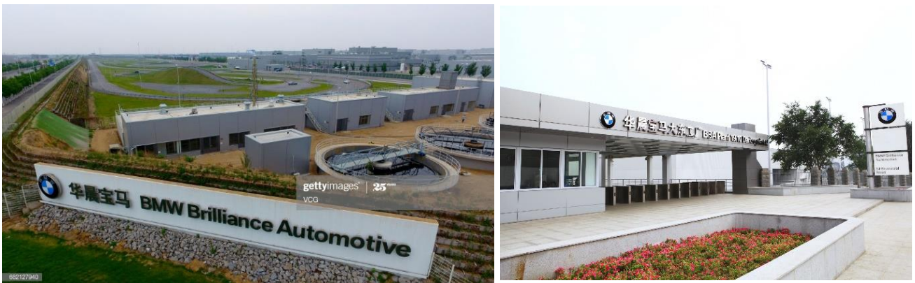
Figure 18: Pictures showing the factory building typology (Source: BMW Group, 2014)
