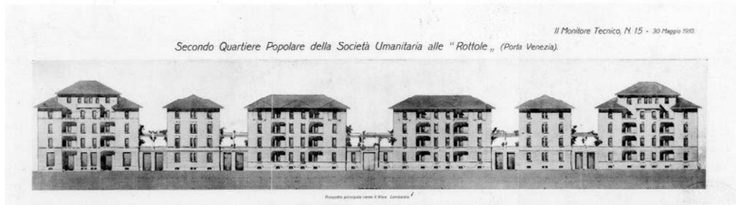
Up: North and south facade.
