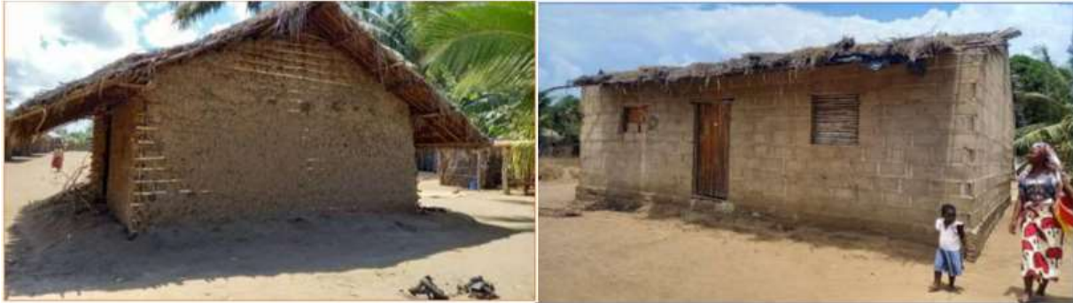
Figure 2-8: Traditional House (on the left) & Semi-Permanent House (on the right).
