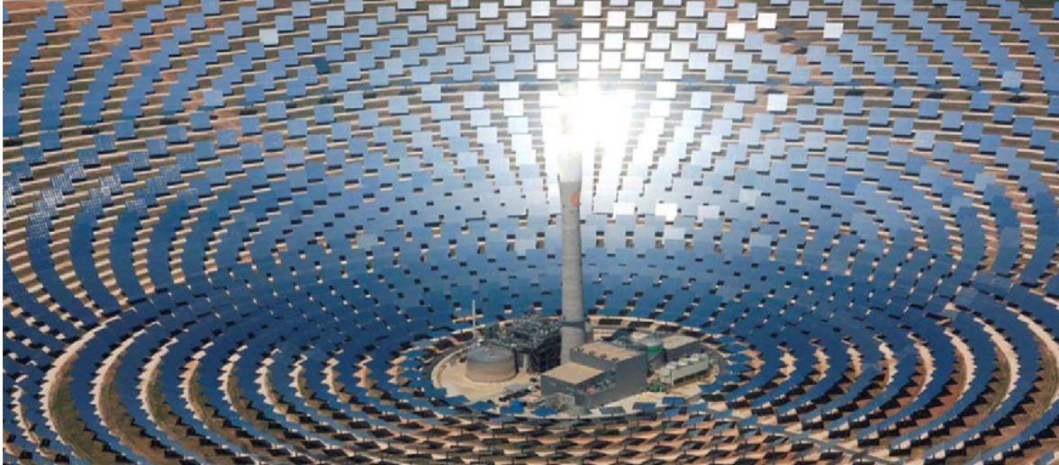
Figure 1.2: View of Gemasolar plant in Spain. With 2650 heliostats, it has 17 MW of electrical power and a net electric production of 80 GWh/year
