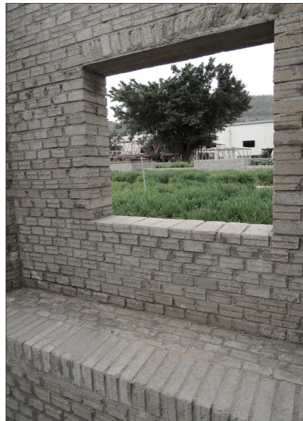
Figure 72. Landscape Framing © Archdaily.com
