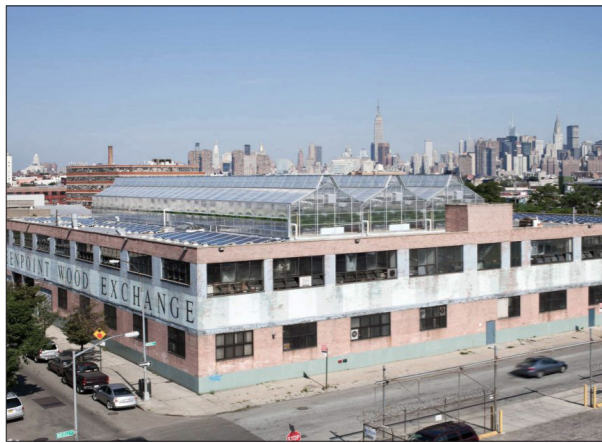
Figure 69. View from Adjacent Rooftop © Gothamgreens.com
