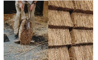
Figure 39. Homegrown: Building a Post-Carbon Future. Photo: Henry Woide.
