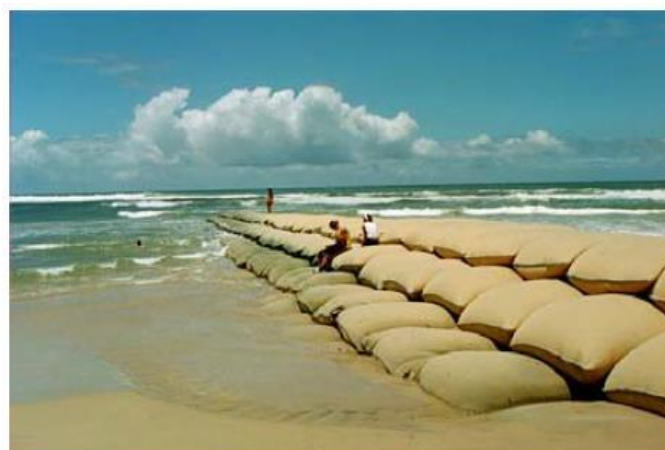
Figure 2.21. Sea Groyne with geotextile containers ( Heibaum, 2006 ).
