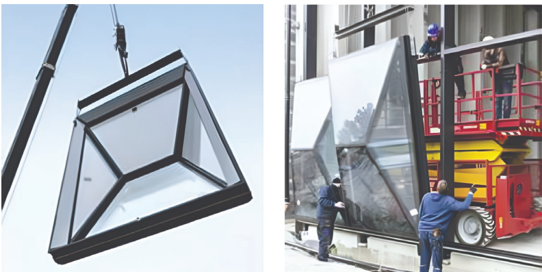
Figure 8.3.3. Unit Prefabrication and Installation of the units on the steel
