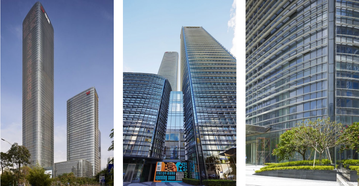
Figure 4.3: Shenzhen Zhongzhou Holdings Financial Center showcasing rectilinear glazed façade with insulated units, designed to balance transparency, thermal efficiency, and mixed-use urban integration
