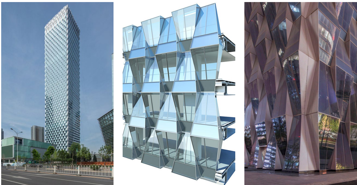
Figure 4.4: Beijing Greenland Center parametric façade modules with prismatic trapezoidal geometry, optimized through digital modeling to enhance self-shading, energy efficiency, and architectural dynamism.
