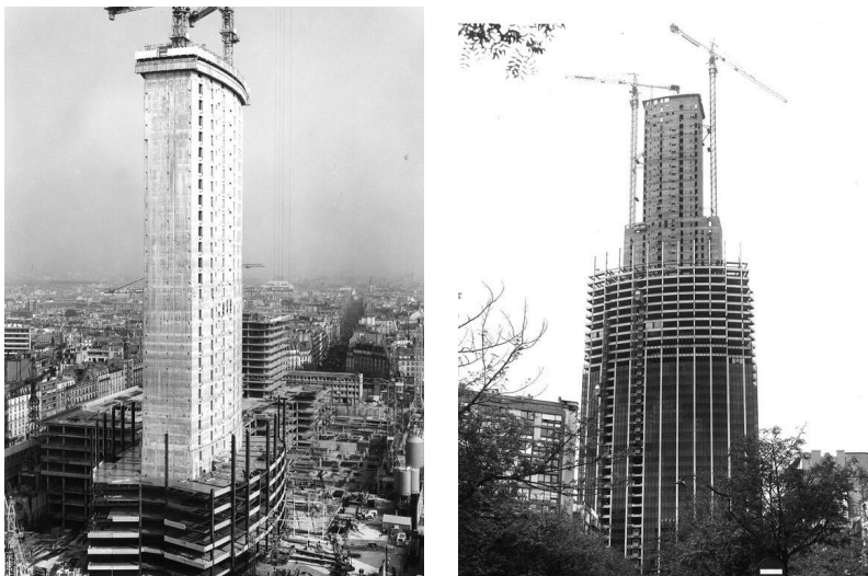
Figure 8.4.1. Montparnasse construction site
