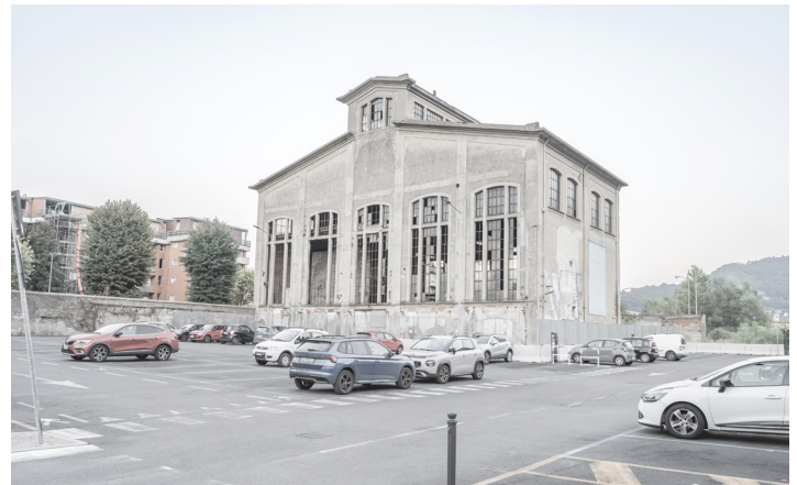
12 | Santarella Thermal power building of the dyeing industry
