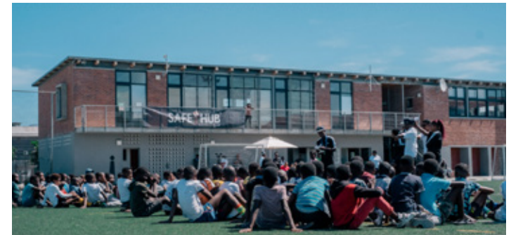
Figure 48: VPUU Medium Active Box: Safe Hub and Resource Centre at Nyanga Junction serving Gugulethu and Manenberg.
