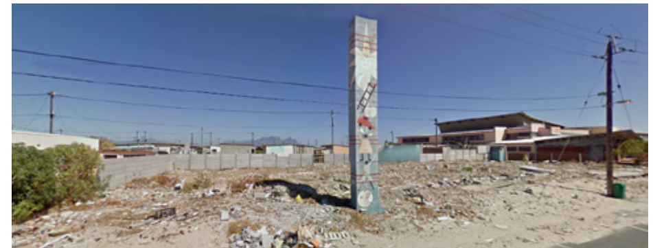
Figure 53: Current condition of site - Daycare destroyed in 2009
