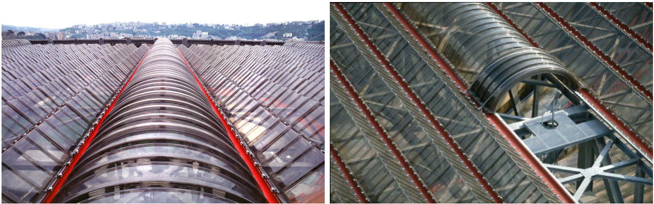
Figure 4.2: Diego Armando Maradona Stadium Roof [34].
