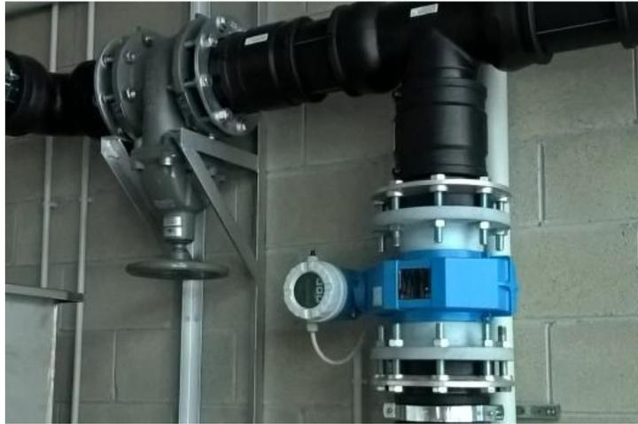
Figure 2.7. Guillotine valve and flow meter.
