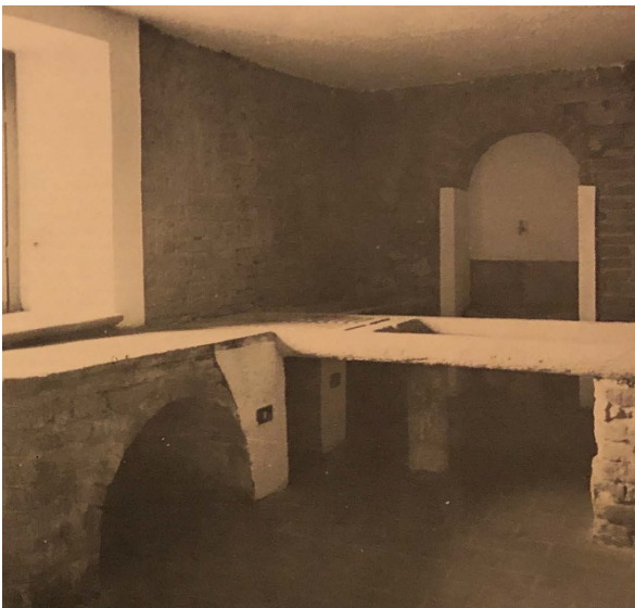
Picture 27. Room 1.14 after the restoration
