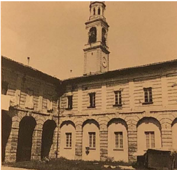
Picture 19. Corridor 1.08 before restoration
