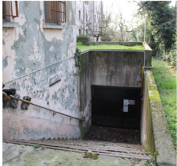
Picture 46. Room 1.41 entrance
