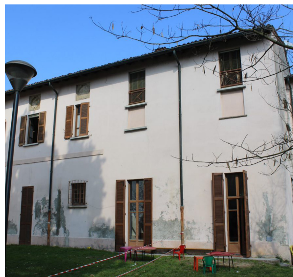
Picture 66. South façade part
