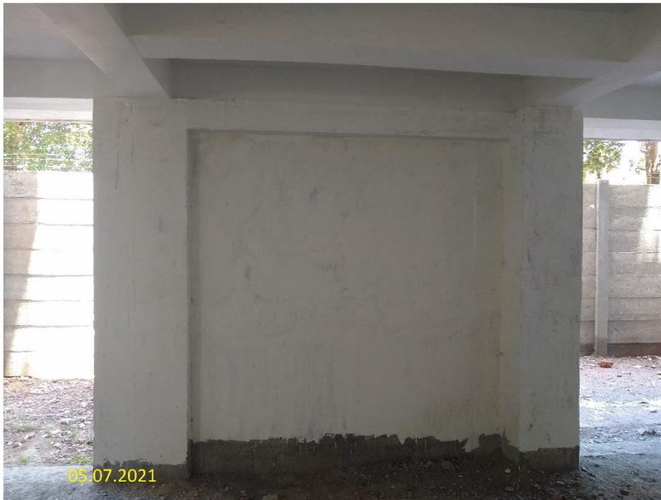
Figure.53. Shear wall and Jacketed column
