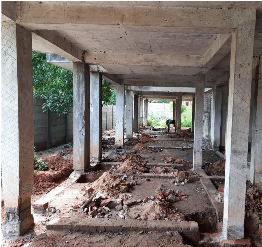
Figure.38. Preparation of column's surface
