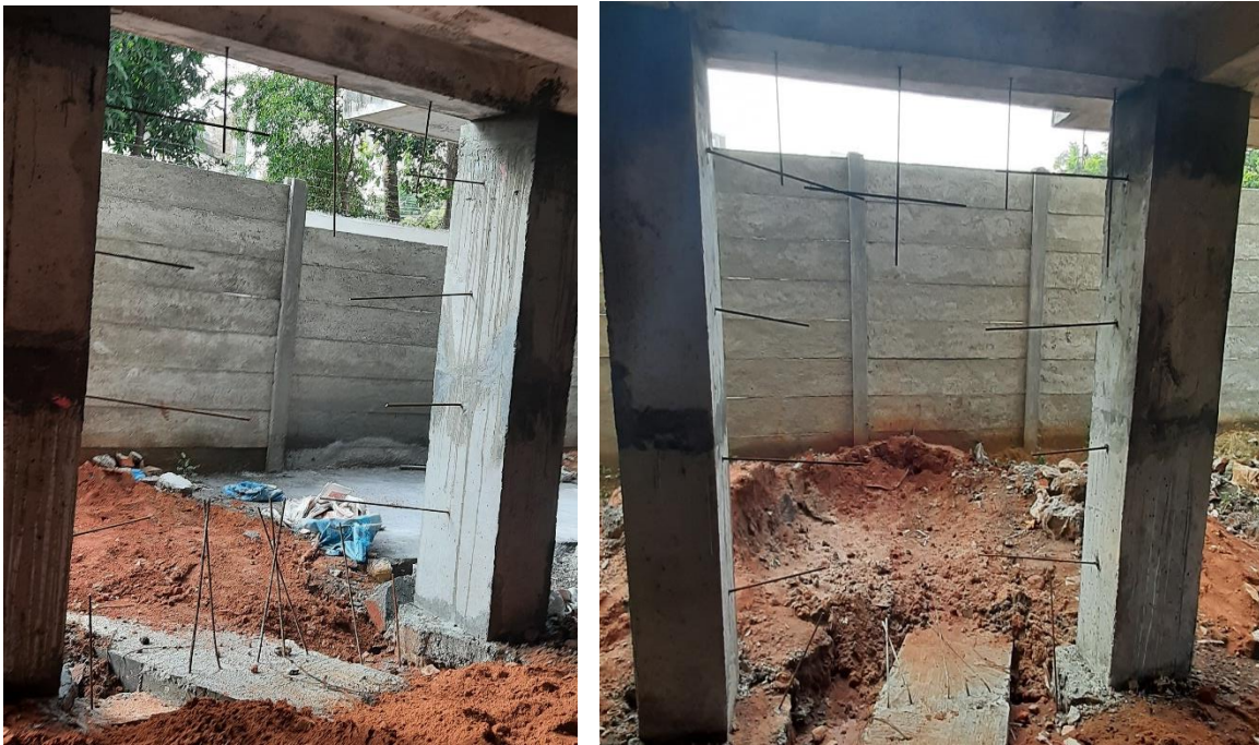
Figure.44. Dowels bar placing
