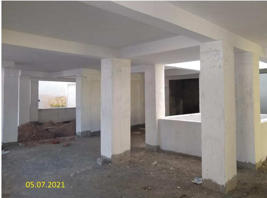
Figure.52. Jacketed Columns
