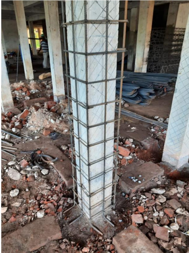
Figure.39. Provision of longitudinal reinforcement
