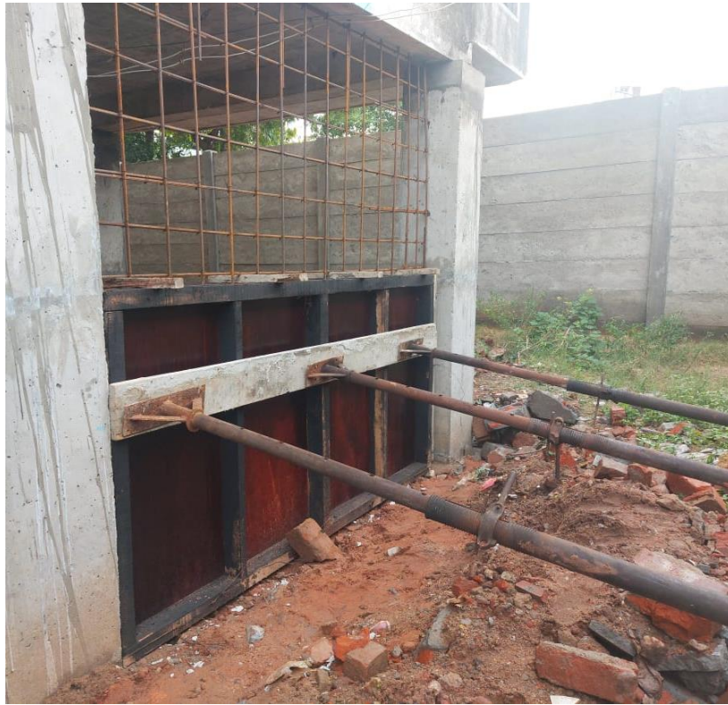
Figure.46. Shear wall shuttering and support
