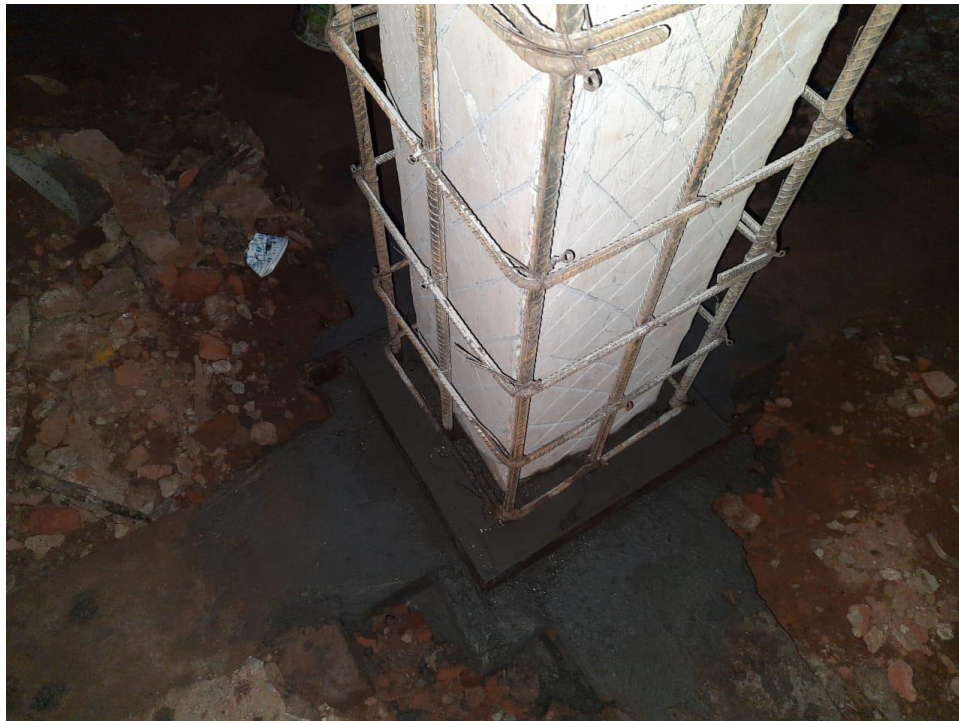
Figure.41. Preparation of column's shoe
