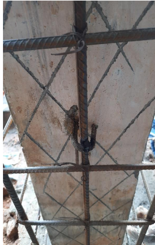
Figure.40. Provision of shear key
