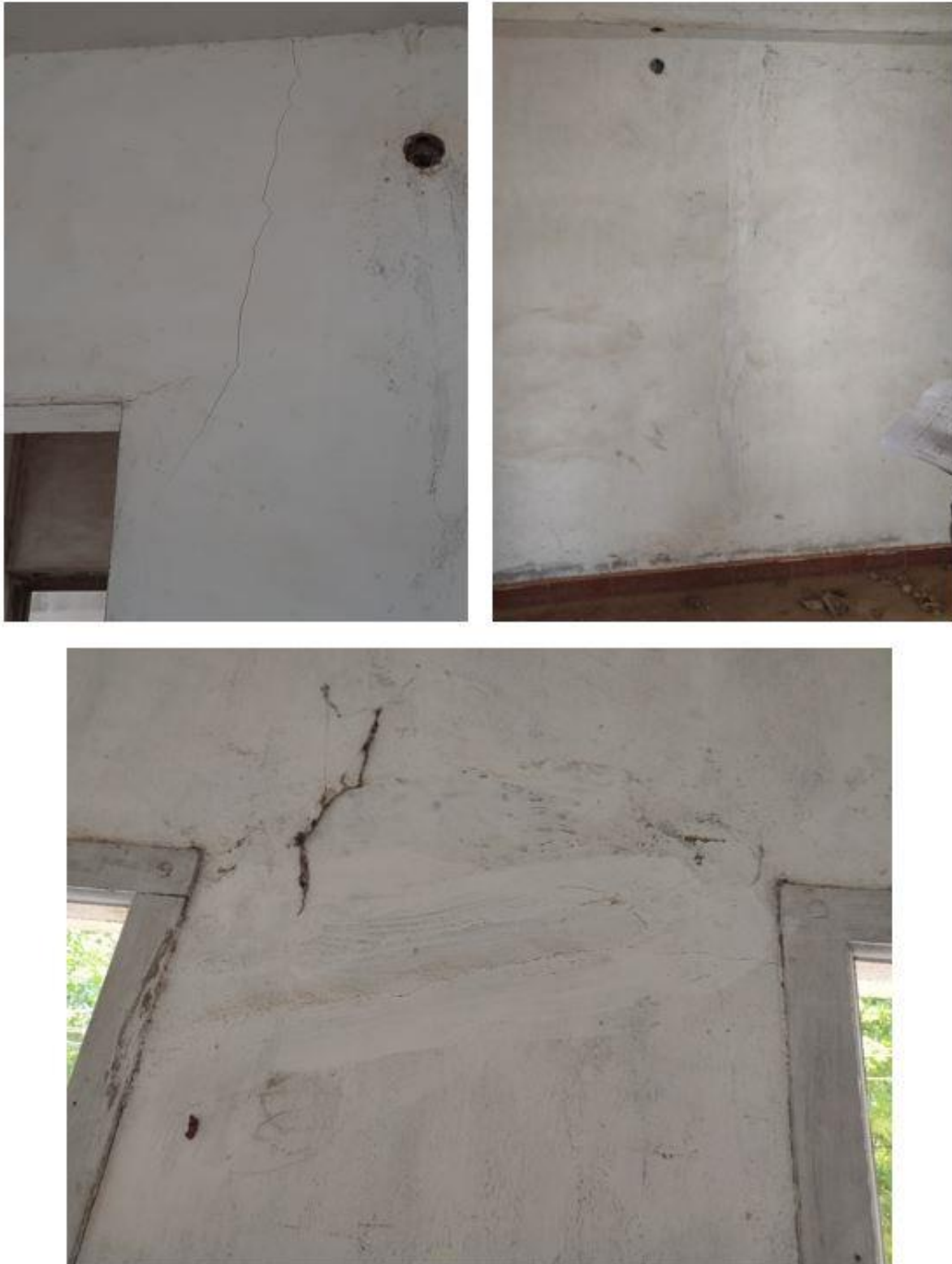
Figure.16. Cracks on the brick wall due to change in climatic conditions
