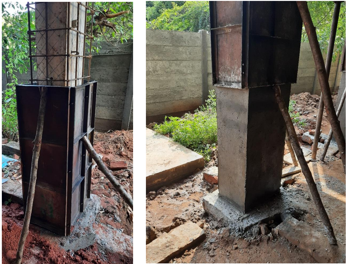
Figure.42. Installation of Formwork
