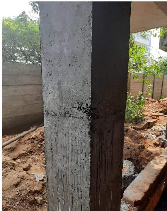
Figure.43. Retrofitted Column
