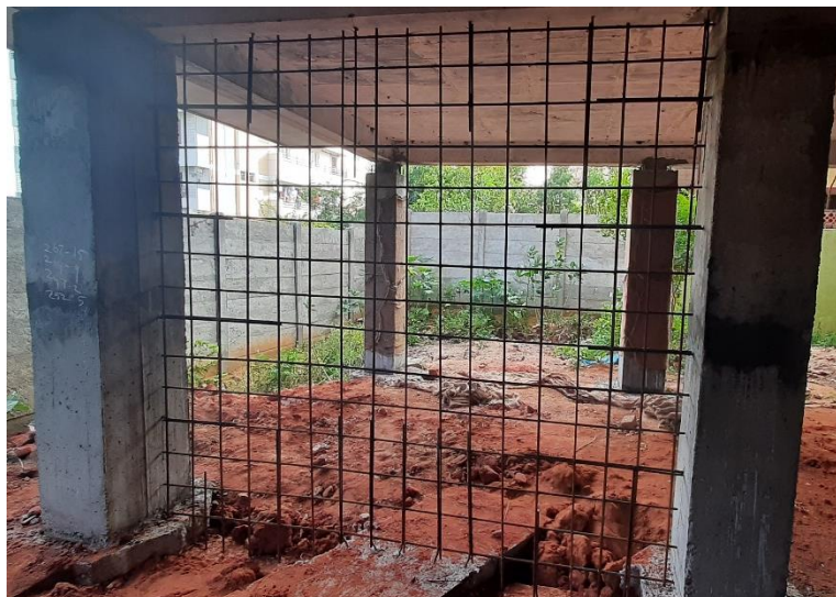
Figure.45. Provision of Longitudinal and Transverse reinforcement
