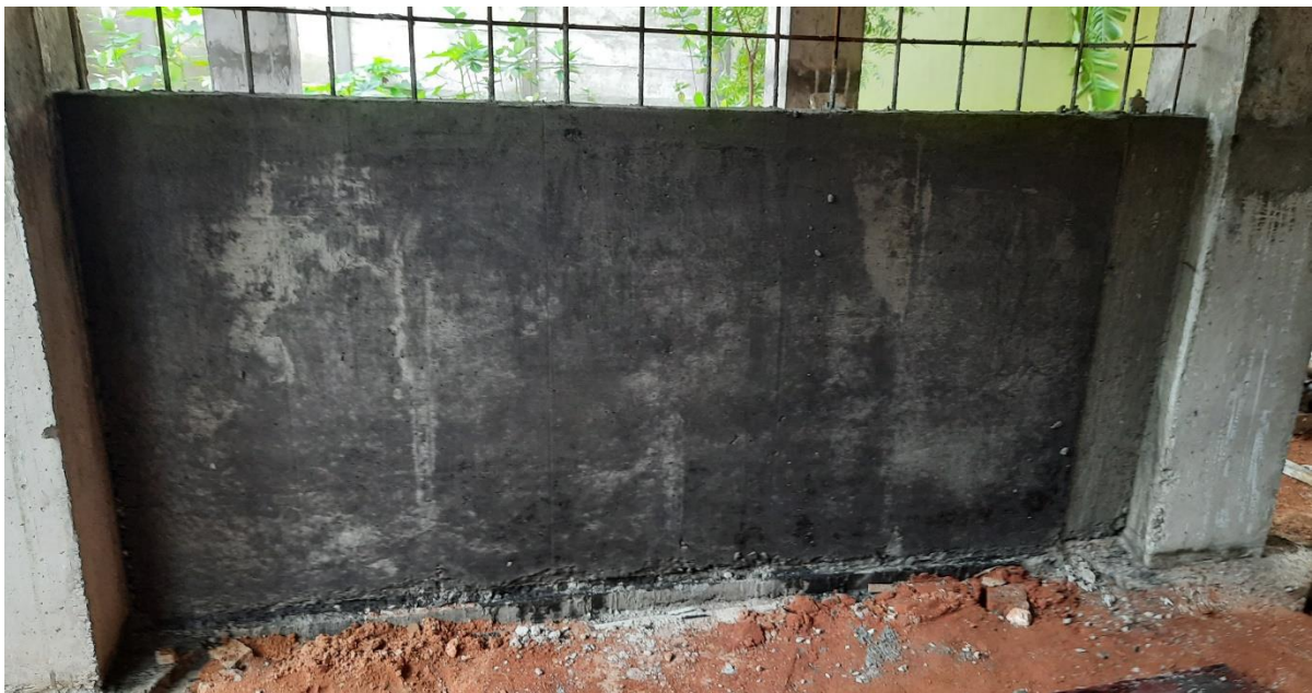
Figure.47. Shear wall concreting
