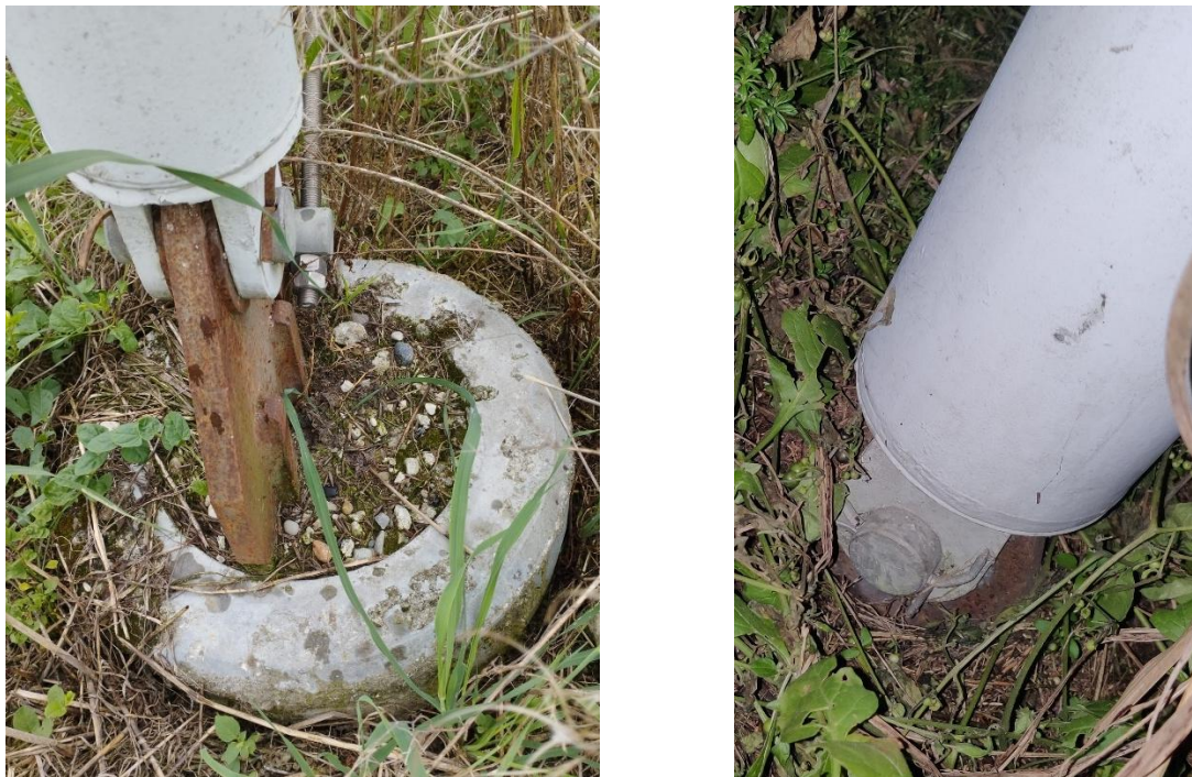
Figure 26 - Foundation of plant of Castelvetro
