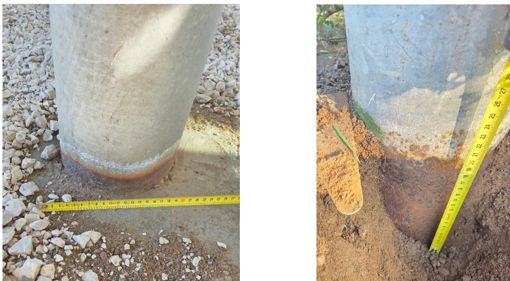
Figure 24 - Foundation and buried part of plant of Pavia
