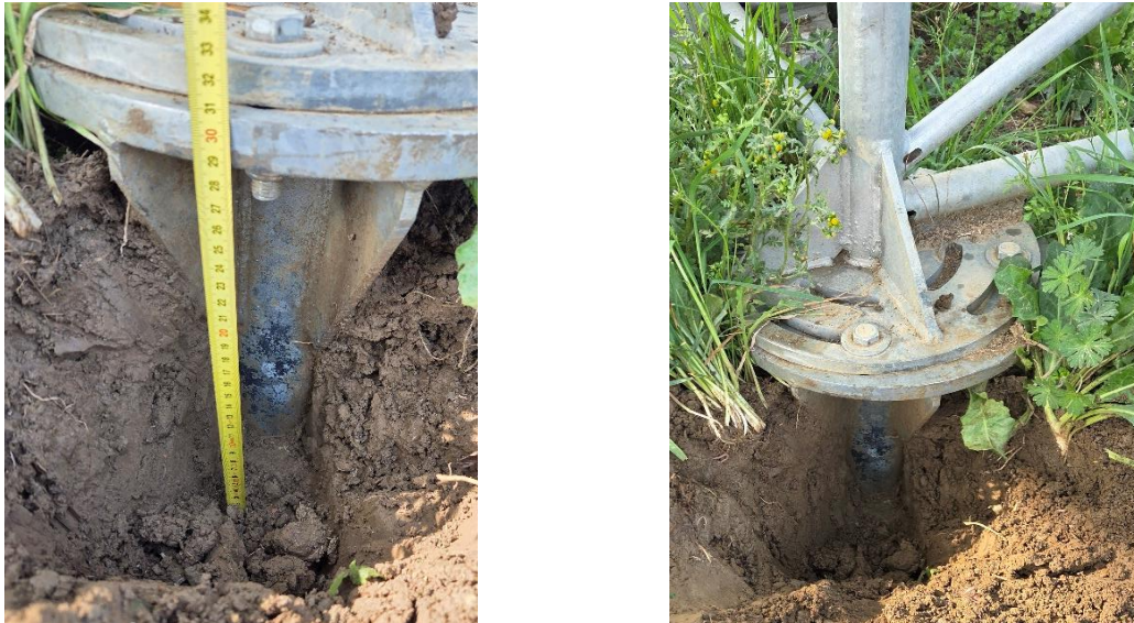
Figure 27 - Buried part of plant of Piacenza
