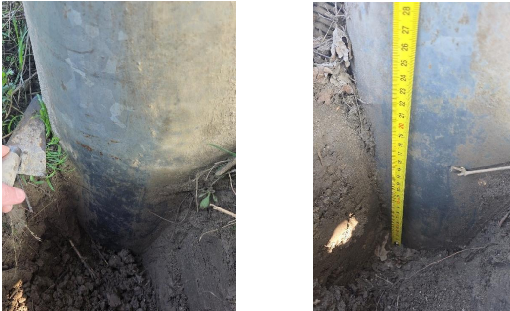
Figure 25 - Buried part of plant of Rovigo
