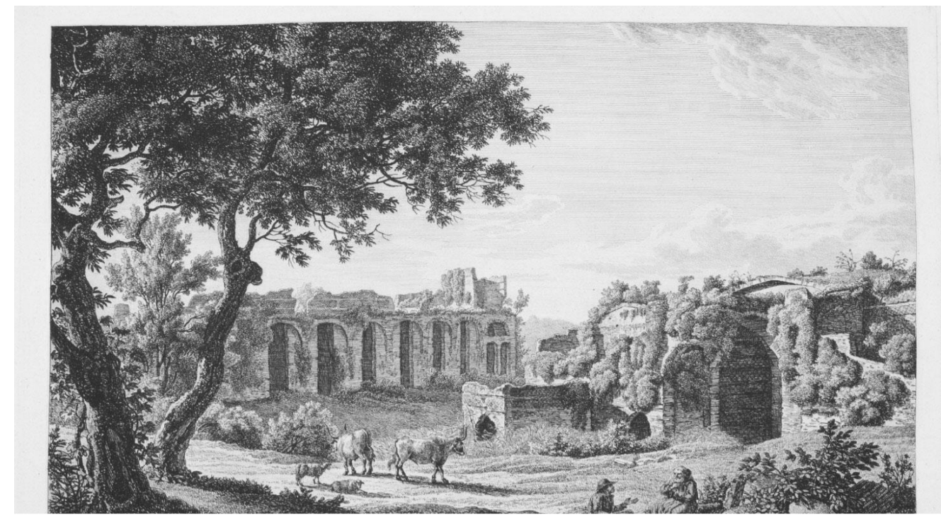
It and the small baths next to it were built after the establishment of the baths of Helioaminus and belong to the extension phase of the villa. It is situated on the south-east side of the Pecile, and its main structure is of brick, with rooms covered with vaulted ceilings.
