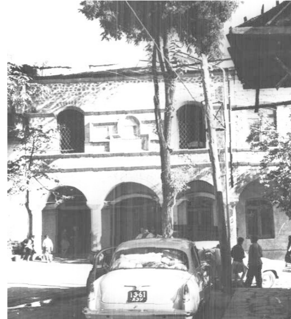
Figure 65: Photo of the entrance. 1977
