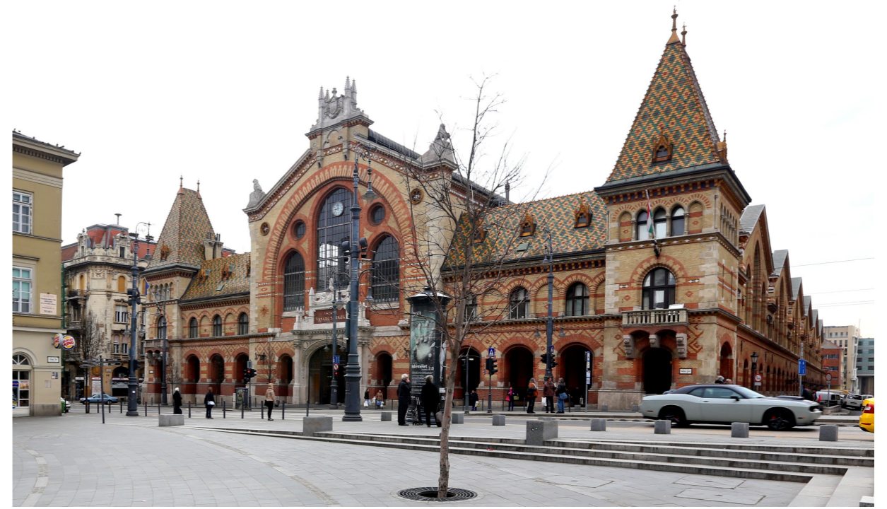
Figure 34: Great Market hall. Adaptation of the building to community requirements, while preserving the identity of the building. 1990s
