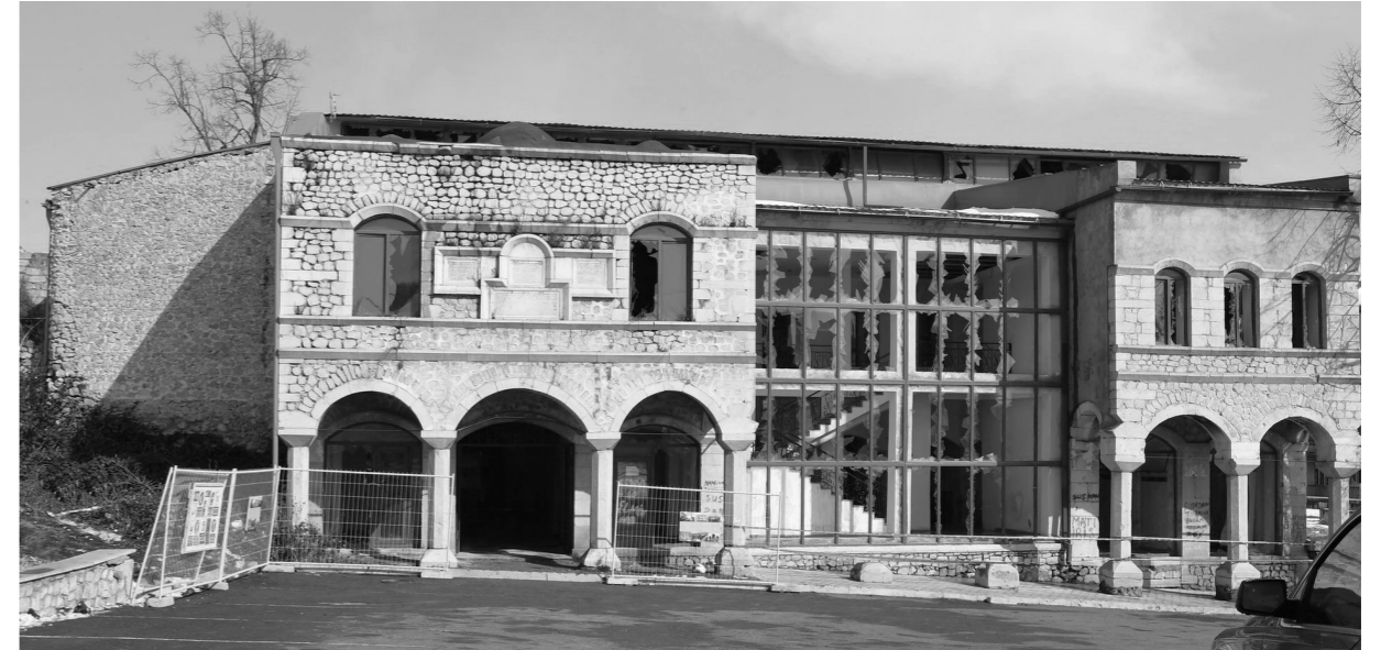
Figure 72: Front view of caravanserai in 2021
