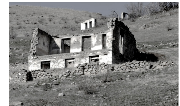
Figure 56: Private house Amirkhanli. Zangilan
