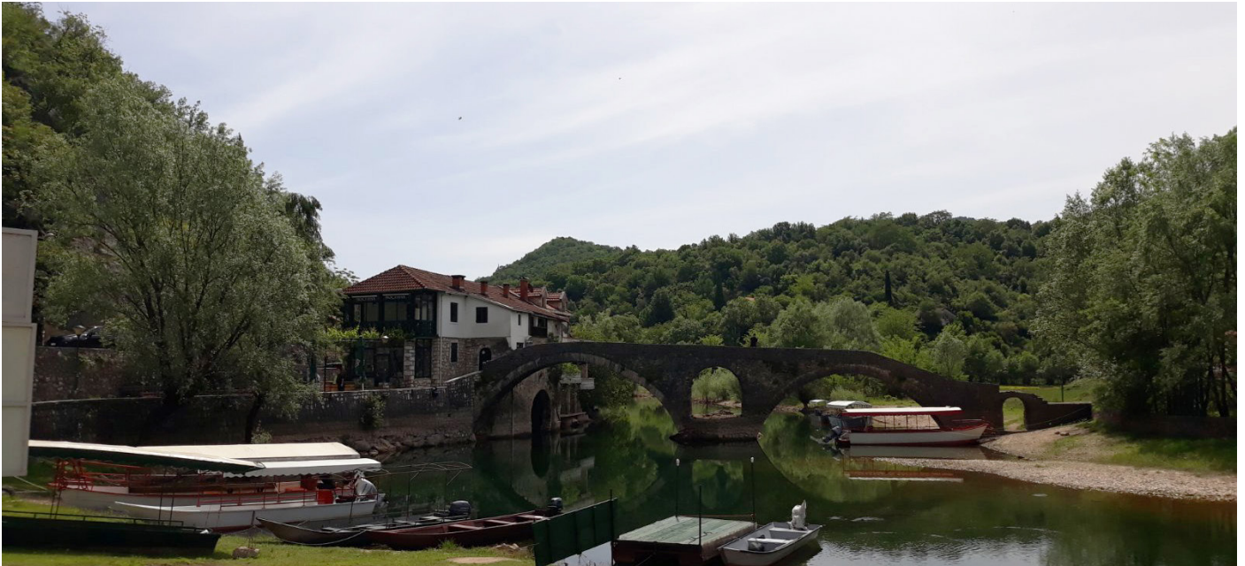
Figure 33: Rijeka Crnojevica, old bridge.
