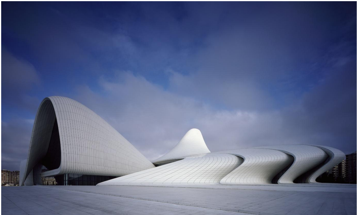
Figure 2.13: Heydar Aliyev Centre external view
