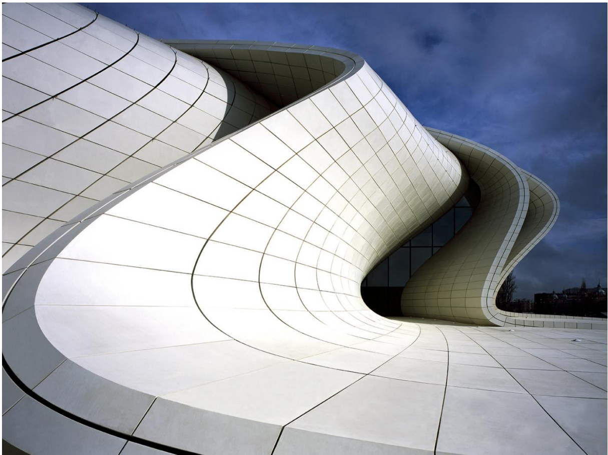
Figure 2.14: Heydar Aliyev Centre close-up faced cladding
