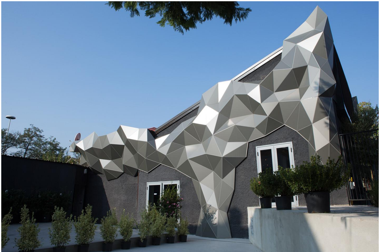
Figure 2.7: Post office external façade
