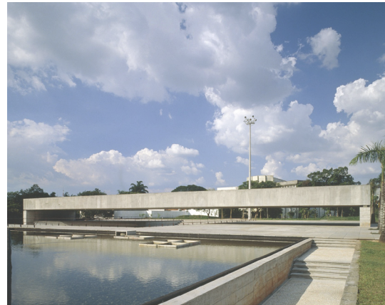
Fig. xx: Picture of the reinforced concrete slab of the Brazilian museum of Sculpture
