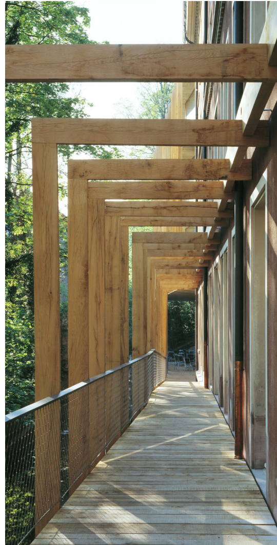
Fig. xx: View of the walkway
