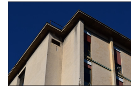
Fig. xx: Picture from the North-West angle
