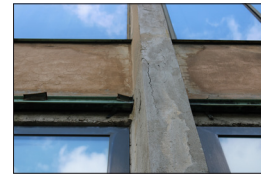
Fig. xx: Close-up of the RC columns
