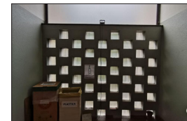
Fig. xx: Interior picture showing vetrocemento
