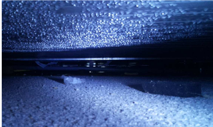
Figure 3.8: Picture taken by the rover during the inspection test. High humidity in the subfloor and unexpected obstacles can be observed. Adapted from [15].
