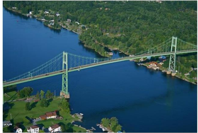
Figure 1.13: Thousand Island Bridge
