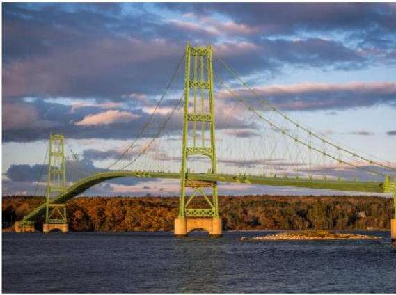
Figure 1.12: Deer Isle Bridge
