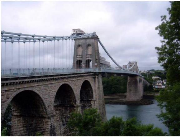
Figure 1.3: Telford's Menai Straits Bridge, Wales
