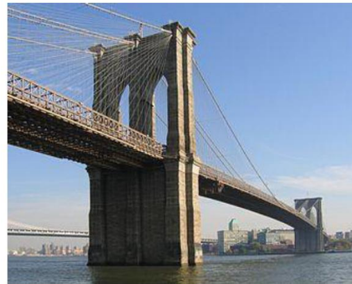
Figure 1.7: Brooklyn Bridge, New York
