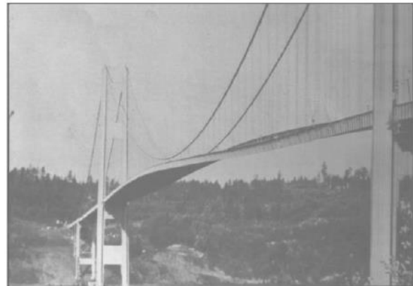
Figure 1.17: Tacoma Narrows Bridge, torsional oscillations
