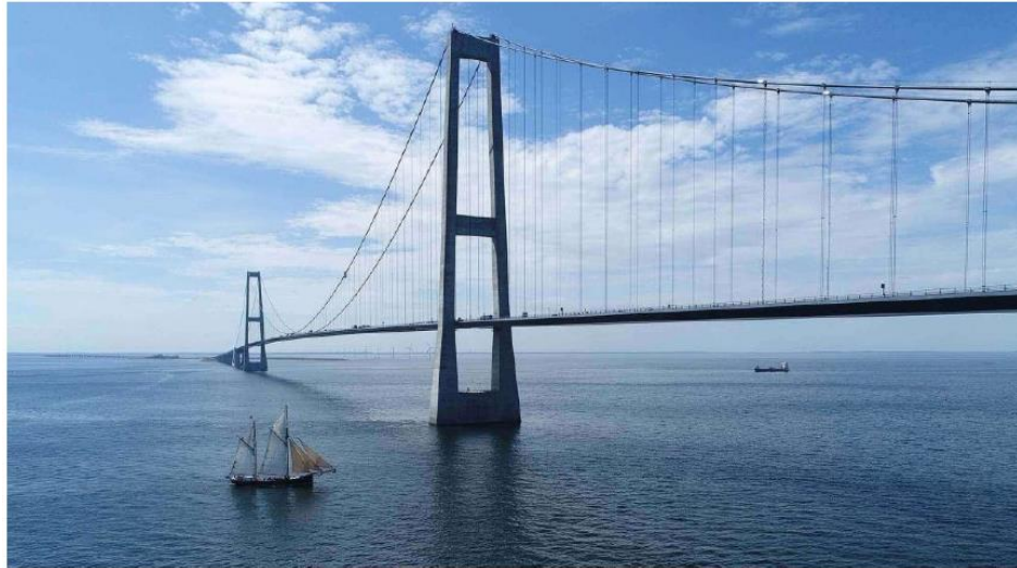
Figure 1.21: The Great Belt Bridge
