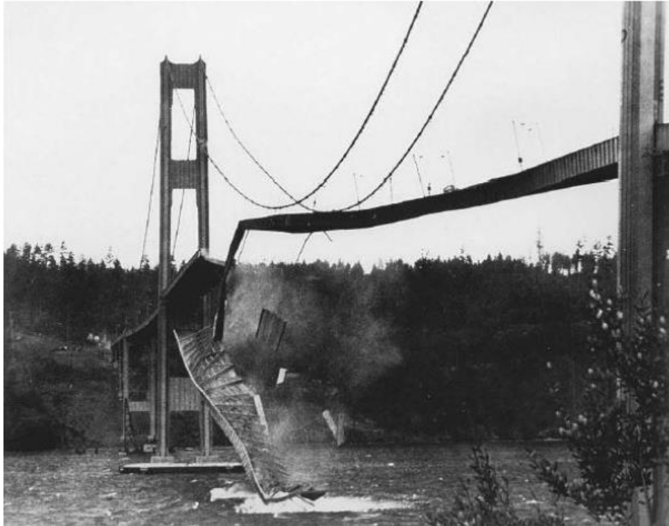
Figure 1.18: Failure of the Tacoma Narrows Bridge
