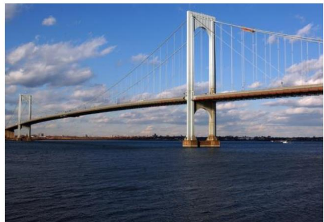
Figure 1.11: Bronx-Whitestone Bridge, New York
