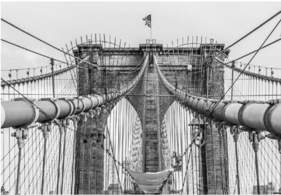
Figure 1.6: Brooklyn Bridge main cables and stays
