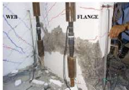
Figure 2.3 Shear failure of one flange end in Ispra Test(Ile & Reynouard, 2005)
