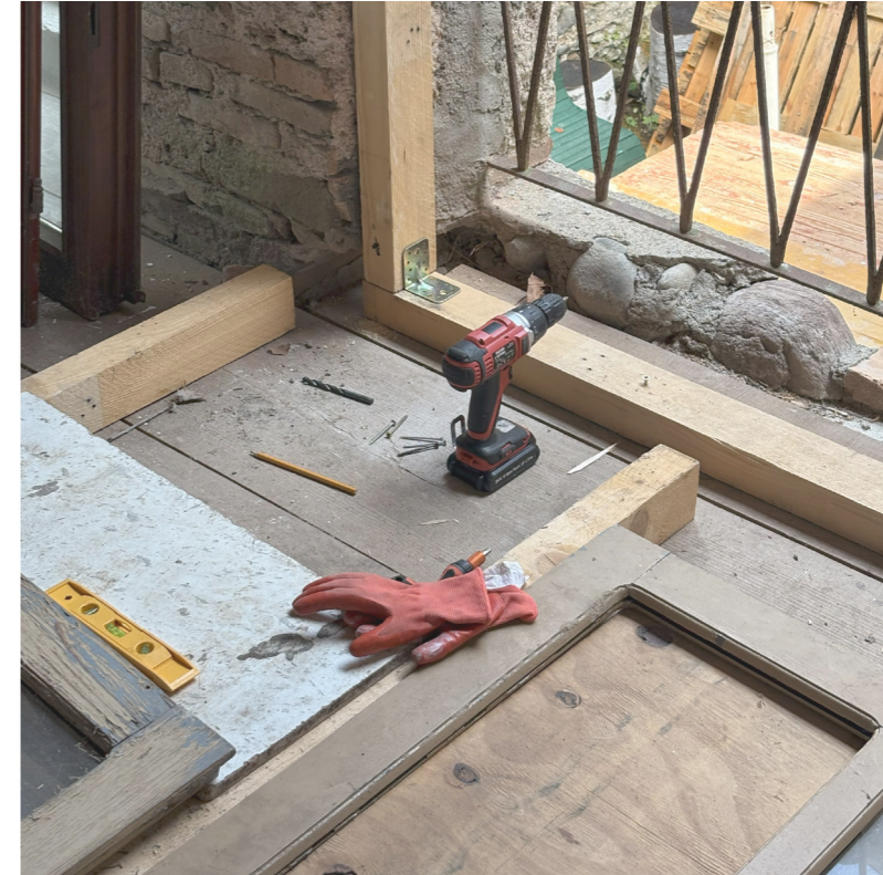
Beginning of the construction
