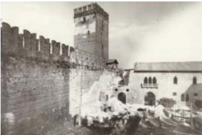
Fig. 04.19: Castelvecchio, before intervention
