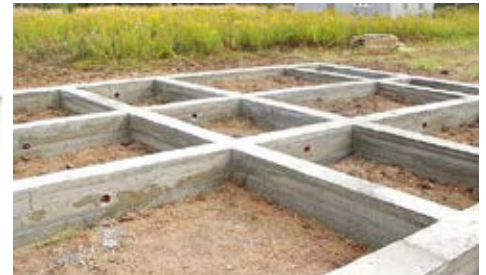
Fig. 04.6: The strip foundation
