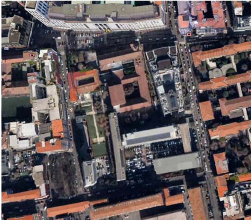
Fig. 01.46: 2020: After the Construction
