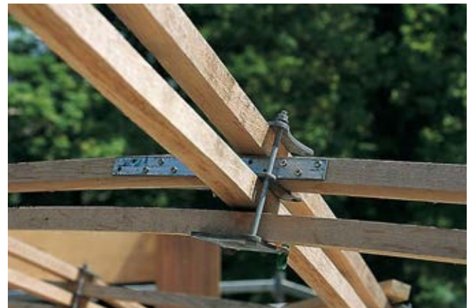
Fig. 04.12: Typical connection showing thinner laths
