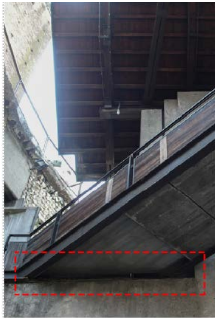
Fig. 04.38: Gap between the existing and new structure, bridge
