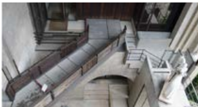
Fig. 04.35: Intervention of the bridge connection
