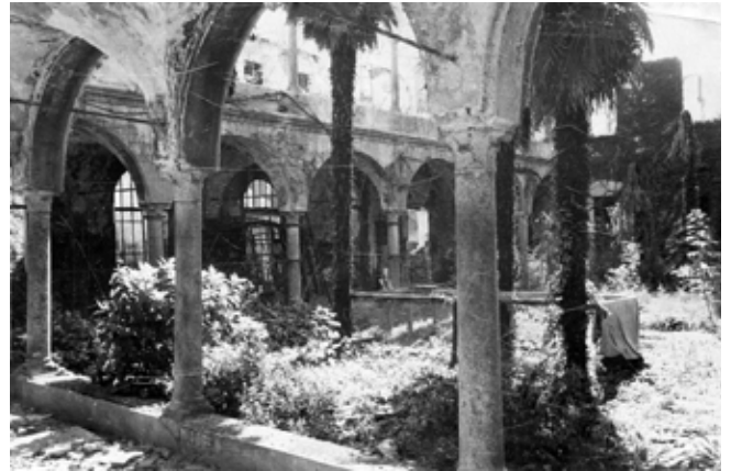
Fig.01.55: A cloister of the Societa Umanitaria after allied raids in 1944
