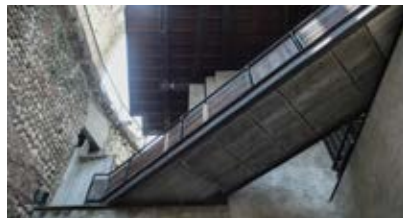
Fig.04.36: Intervention of the bridge connection
