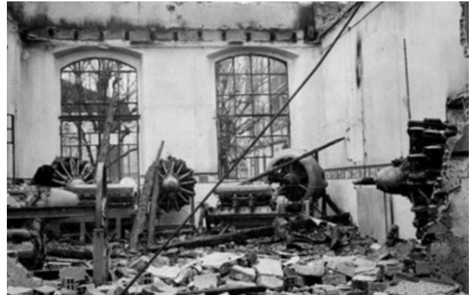
Fig.01.40: Demolished Umanitaria Building
