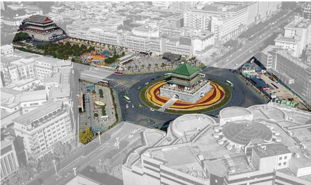
FIGURE 40 THE BIRD VIEW OF BELL & DRUM TOWER PLAZA
