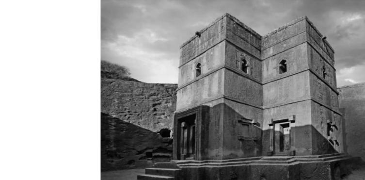
The churches are primarily monolithic as they use the process of carving from rock from ground level down. This requires the excavation of a trench which further develops into the detailing of entryways, Arches, alters, stairs, doors etc.
