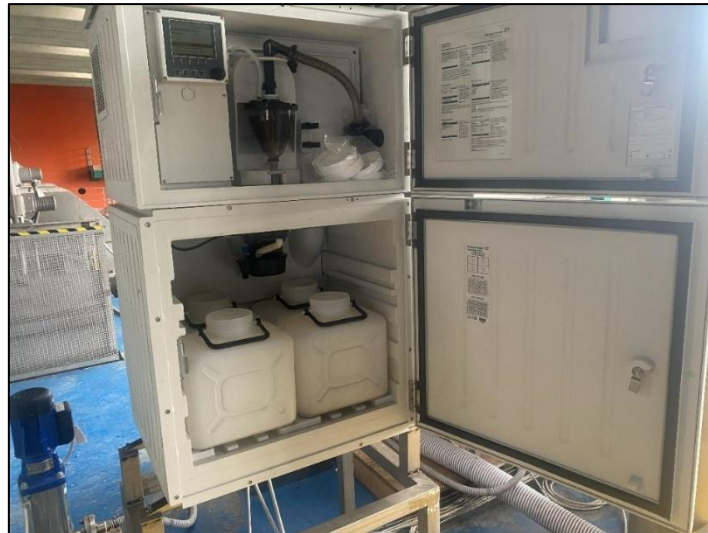
Figure 21: Sampling system (Endress+Hauser Liquistation CSF28)
