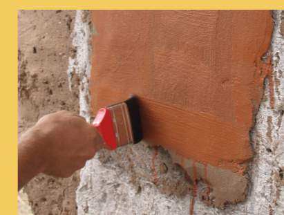
Stabilized loam mortar
