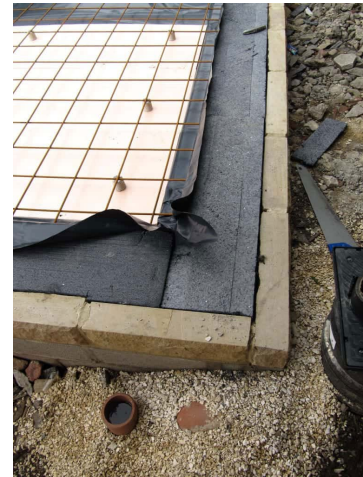
The DPC tray between the wall batts and the EPS insulation cut at an angle
