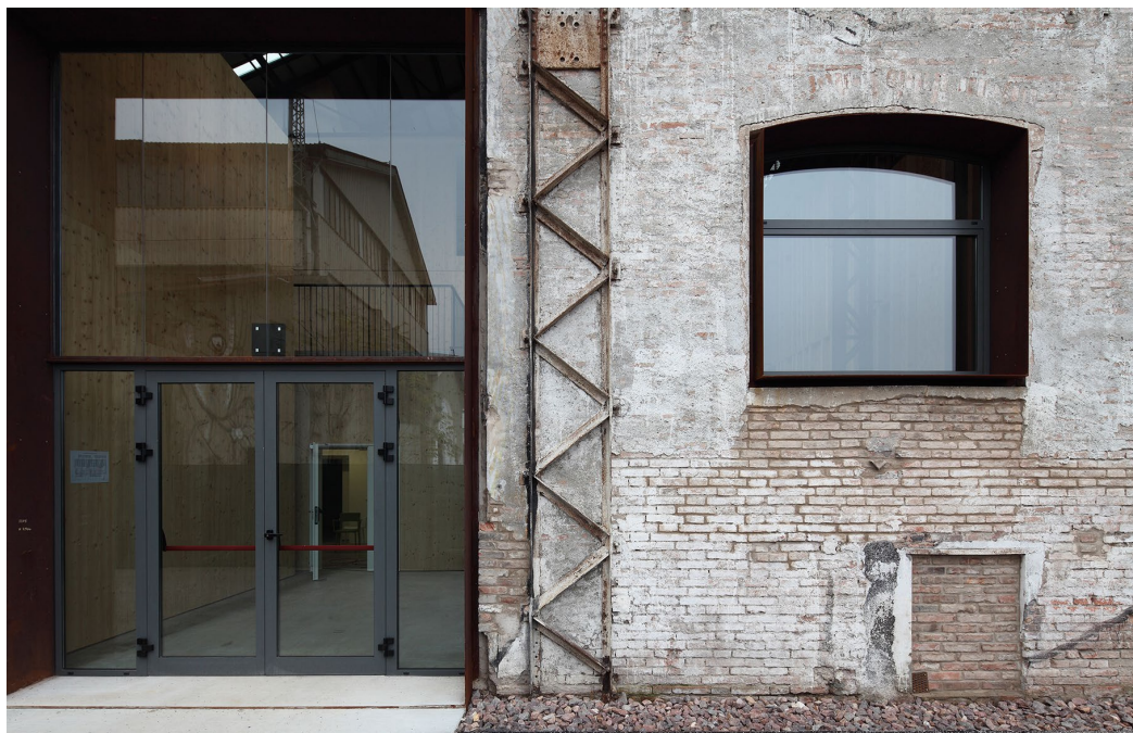
Figure 31 Detail of intervention (source: Archdaily website)
