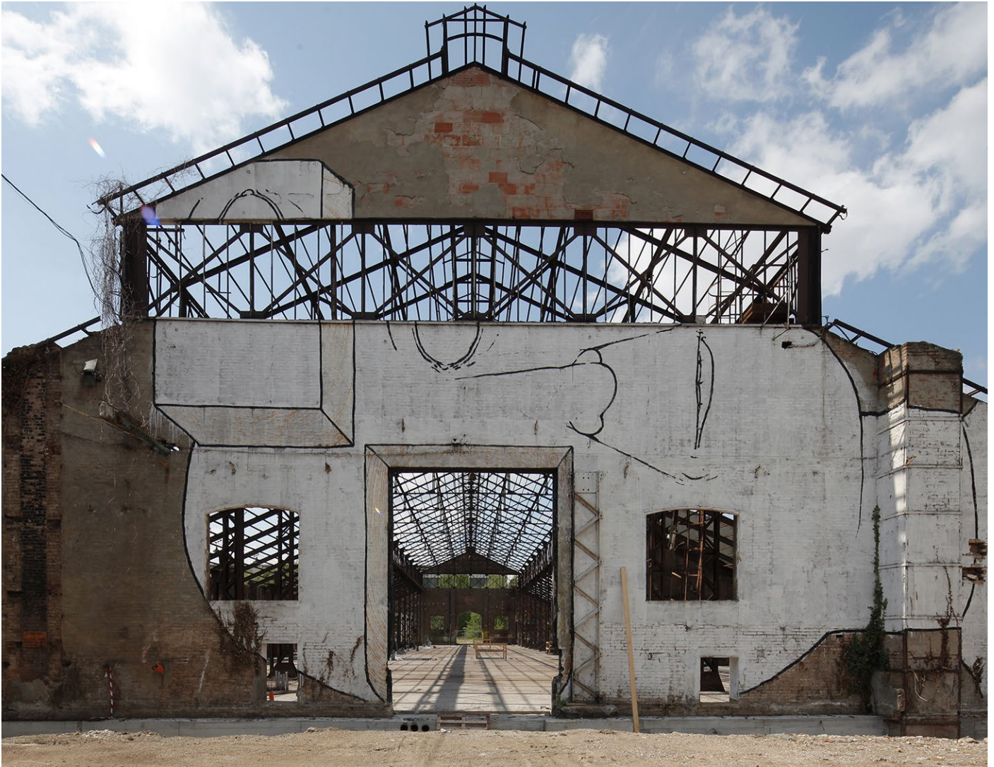
Figure 9 Initial state before renovation process (source: Archdaily website)
