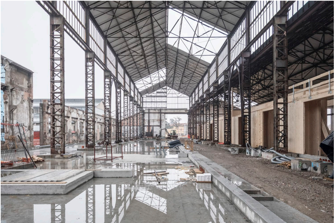
Figure 12 New structure following original shape (source: Archdaily website)
