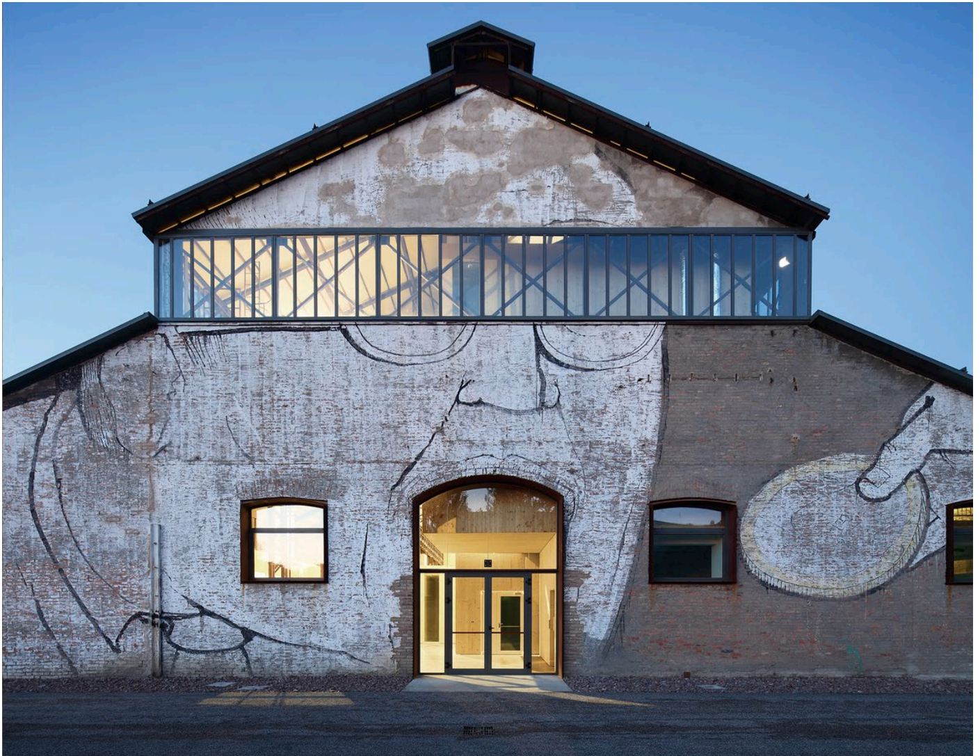
Figure 10 Facade after renovation (source: Archdaily website)
