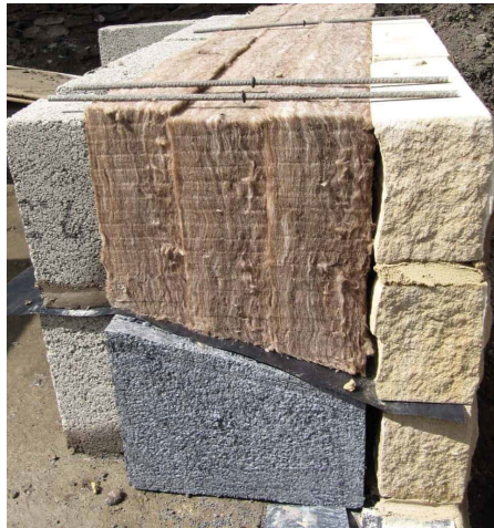
The DPC tray between the wall batts and the EPS insulation cut at an angle
