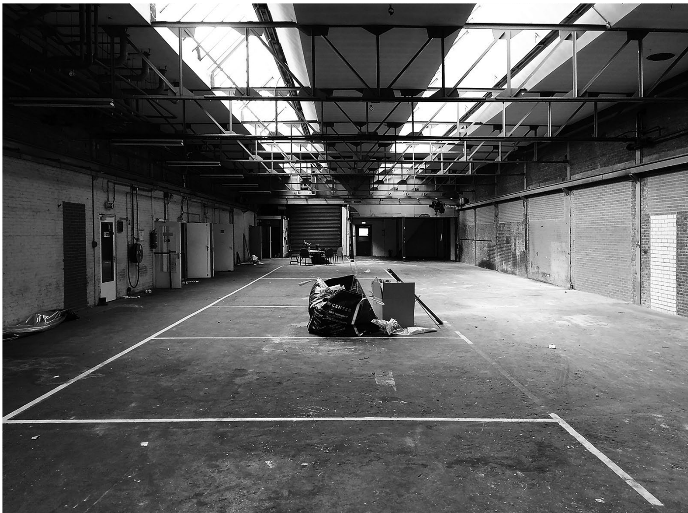
Figure 35 Interior space before intervention showing existing skylights 8
