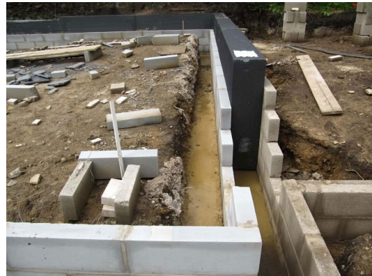
Denby Dale block cavity wall
