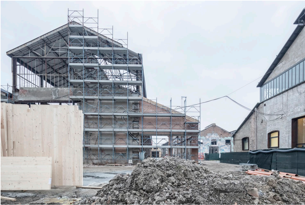
Figure 19 In the process of renovation (source: Archdaily website)
