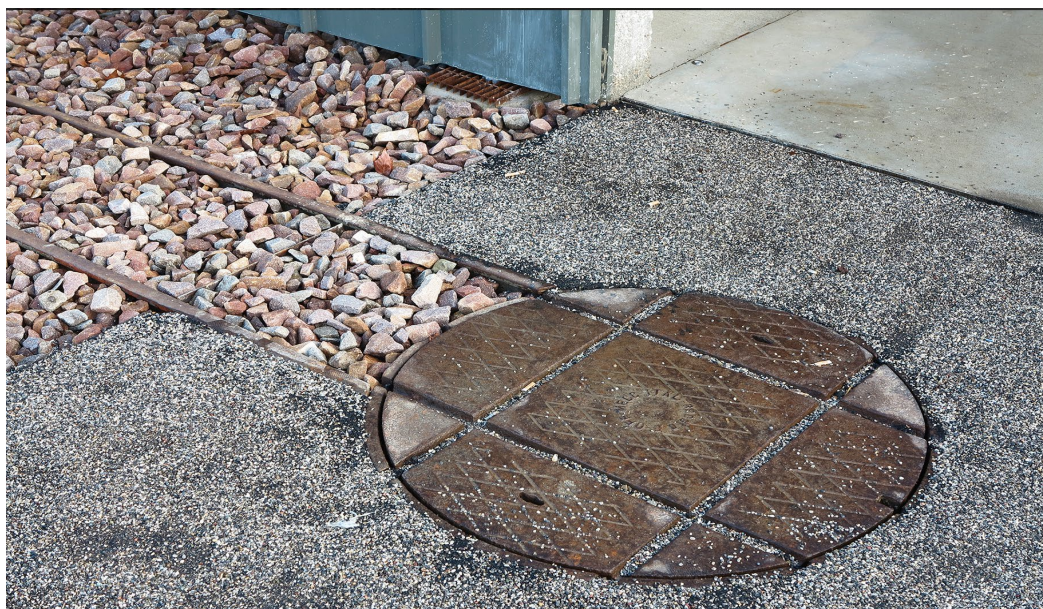
Figure 32 Detail of intervention (source: Archdaily website)
