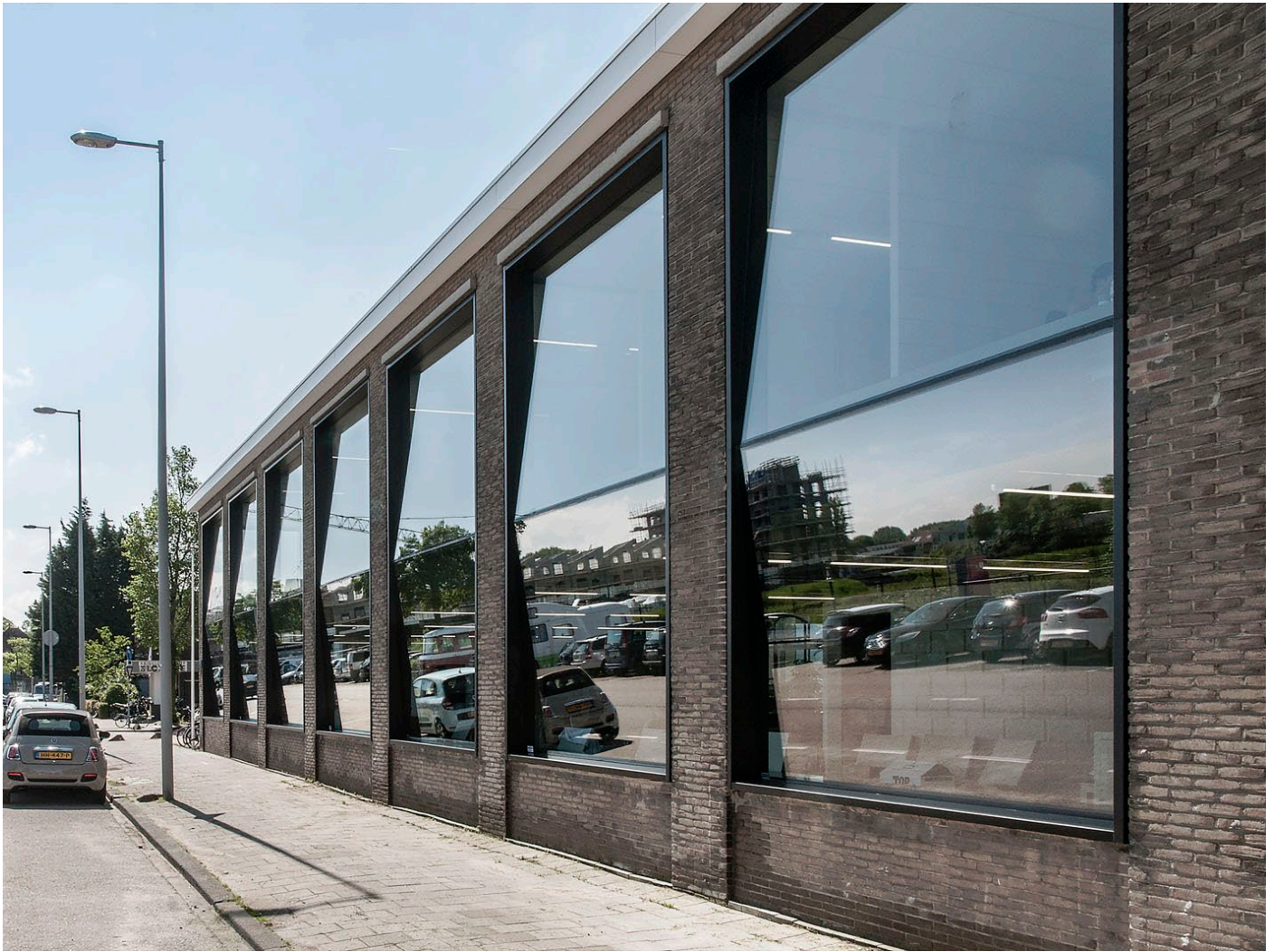
Figure 34 New large openings in the office facade (Source: Archdaily Website)
