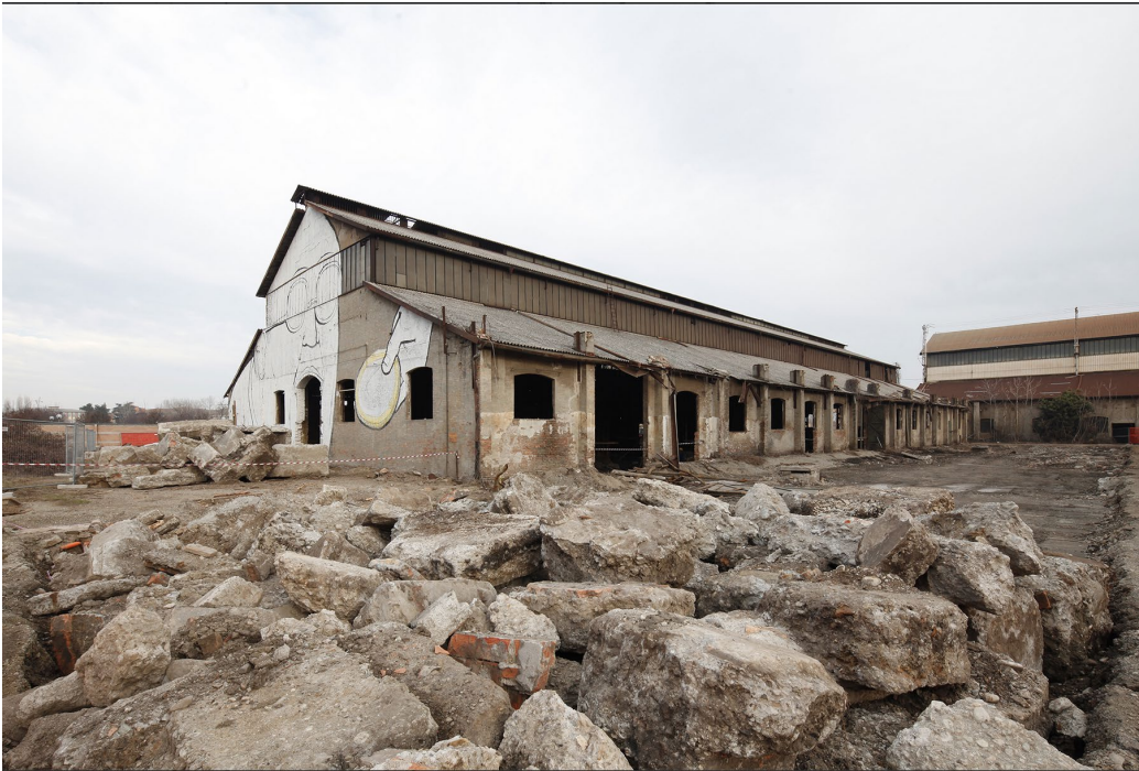
Figure 23 Before intervention (source: Archdaily website)
