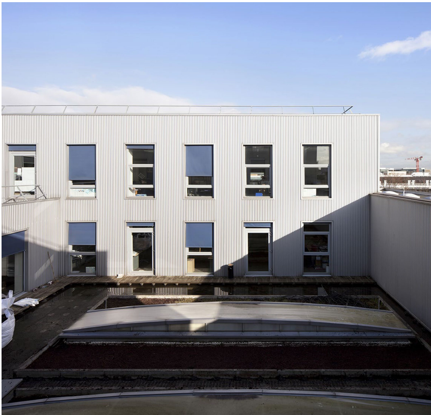
Figure 46 The previous state of the roof (source: Archdaily)
