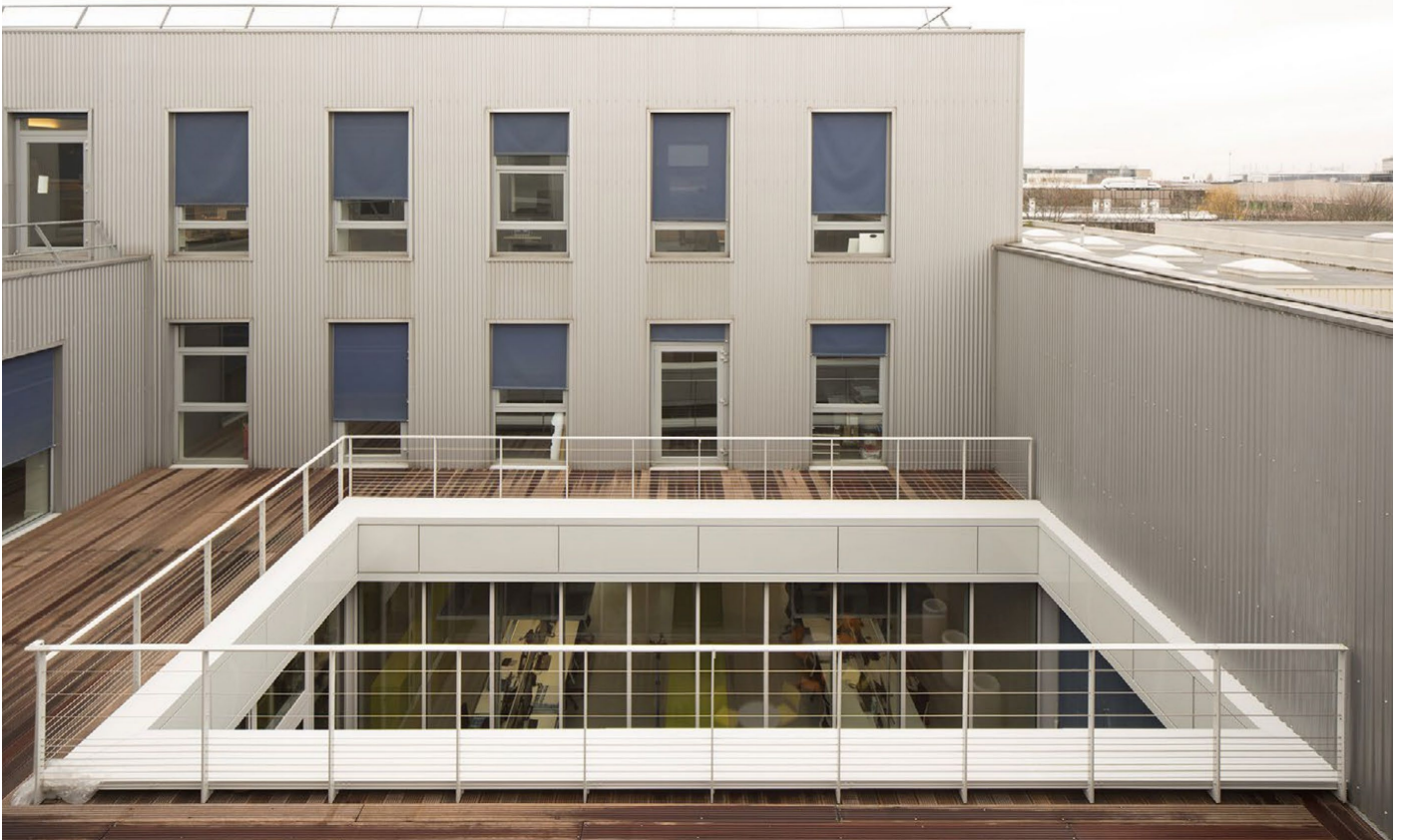
Figure 47 The new patio created inside the existing patio (source: Archdaily)
