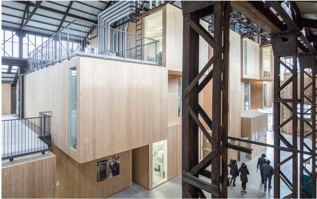
Figure 13 Interior space showing modules (source: Archdaily website)
