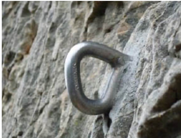
Figure 5 Glue - in bolt fixed in the rock
