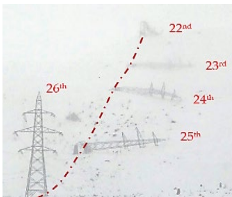
Figure 1: Towers from n22 to n26 after the storm, 2018 (source SwissGrid). Marked in red, the line path, towers n22 to n25 fallen in the perpendicular direction, n22 failed at midheight, the others at the basement; n26 still intact.
