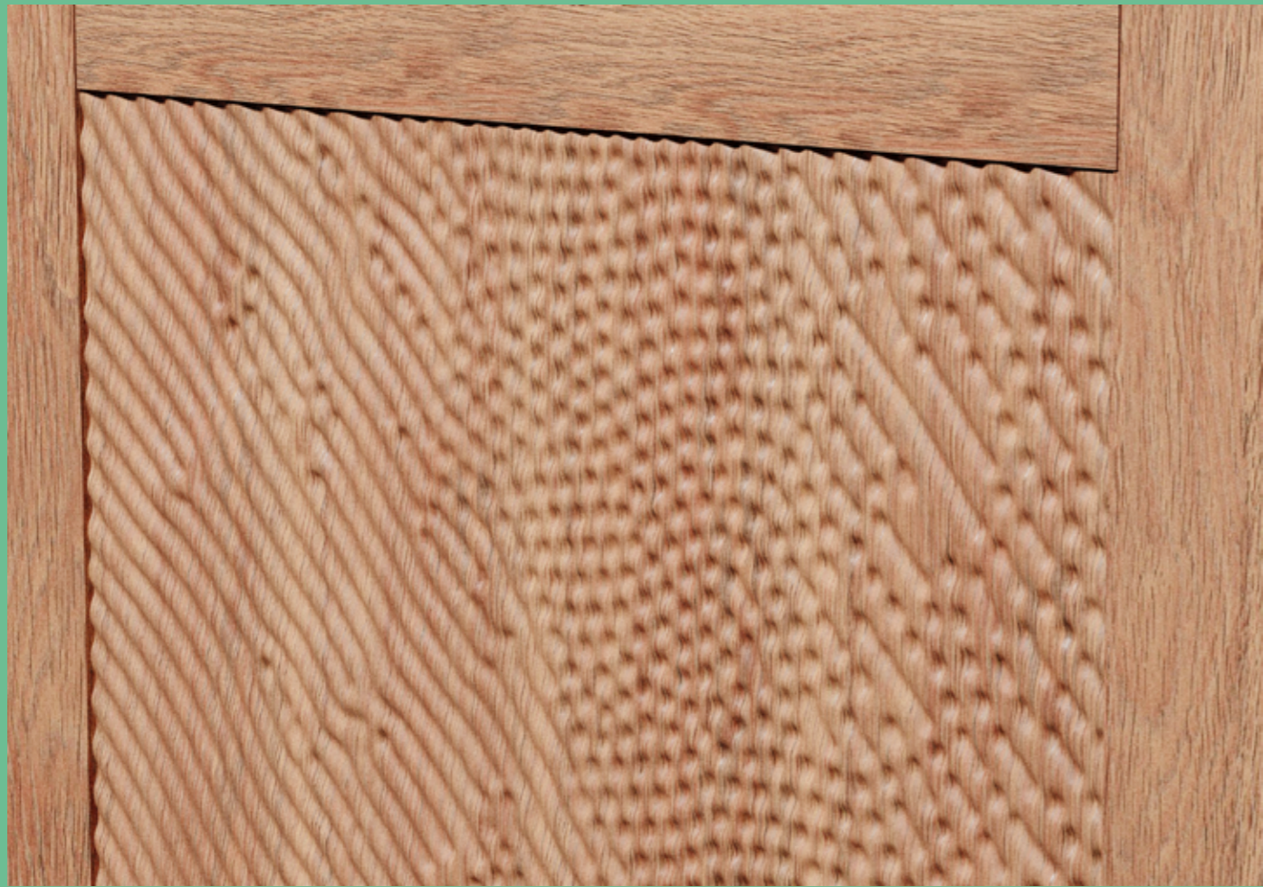
ILL 118 detail of the patterned panel, framed by rails and stiles
