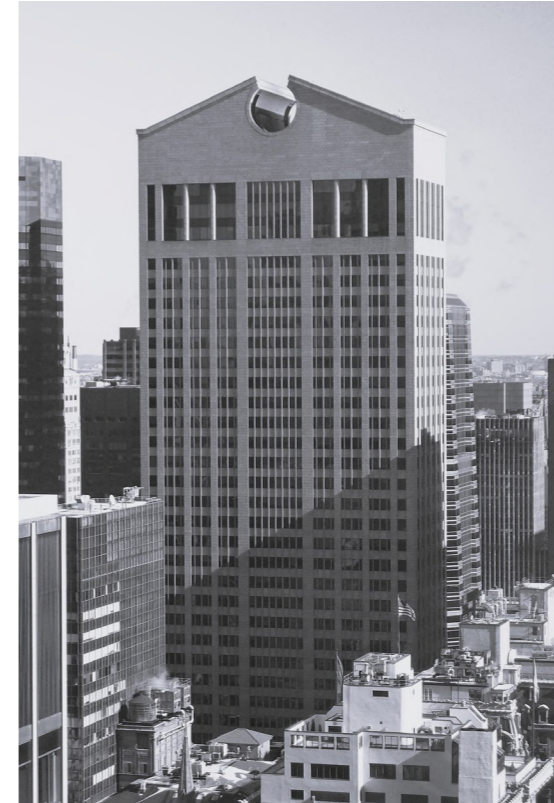
P. Johnson. AT&T. New York, United States. 1983. Available at: www.archdaily.com/611169/ad-classics-at-and-t-building-philip-johnson-and-john-burgee
