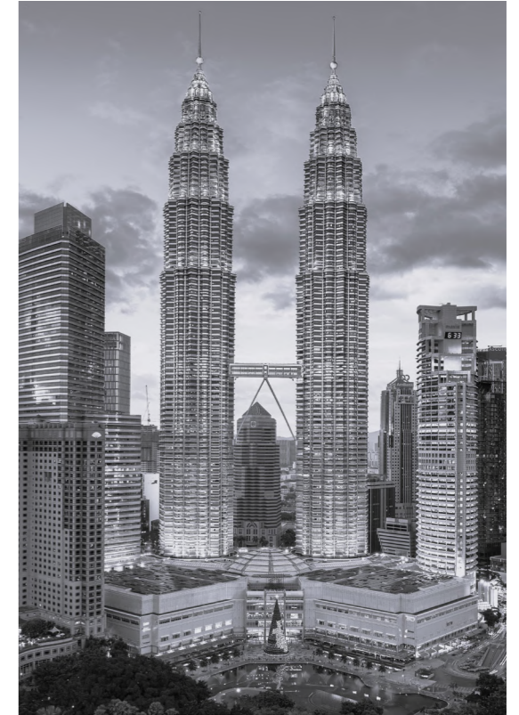
C. Pelli. Petronas Twin Towers. Kuala Lumpur, Malasia. 1999. Available at: https://de.wikipedia.org/wiki/Petronas_Towers
