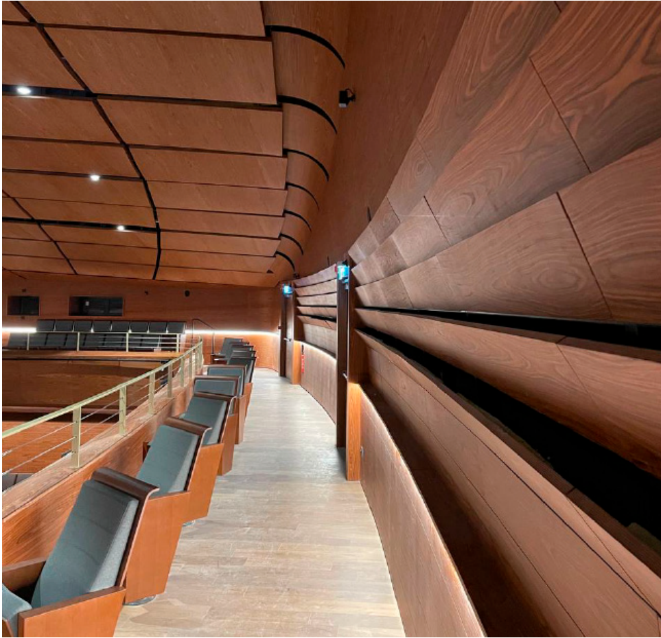
Figure 1.5: Second gallery on the left side of the hall with open pivoting panels.
