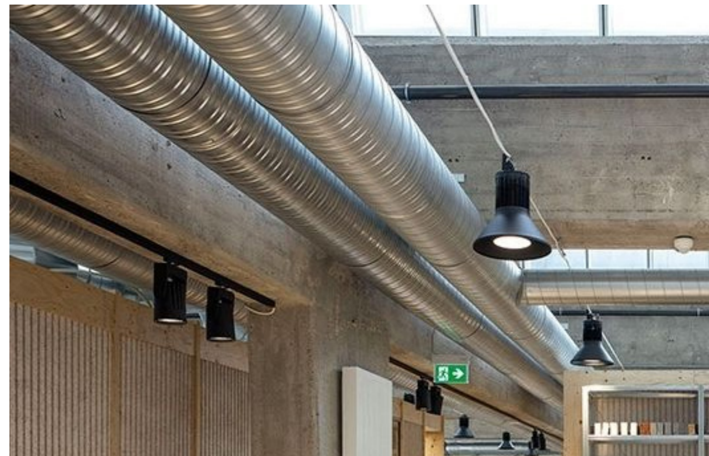
Figure 7.7: Thermax Thermaround Architectural Duct System
