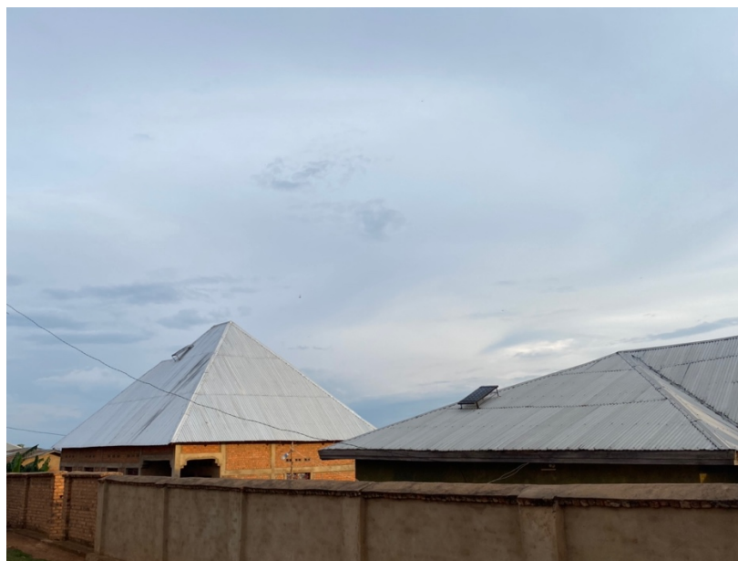
Figure 27:solar home system
