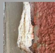
Figure 111: Efflorescence
