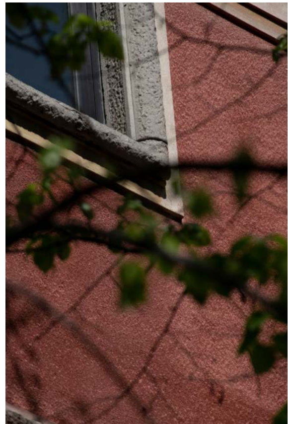
Figure 41: Window moldings on the existing building
