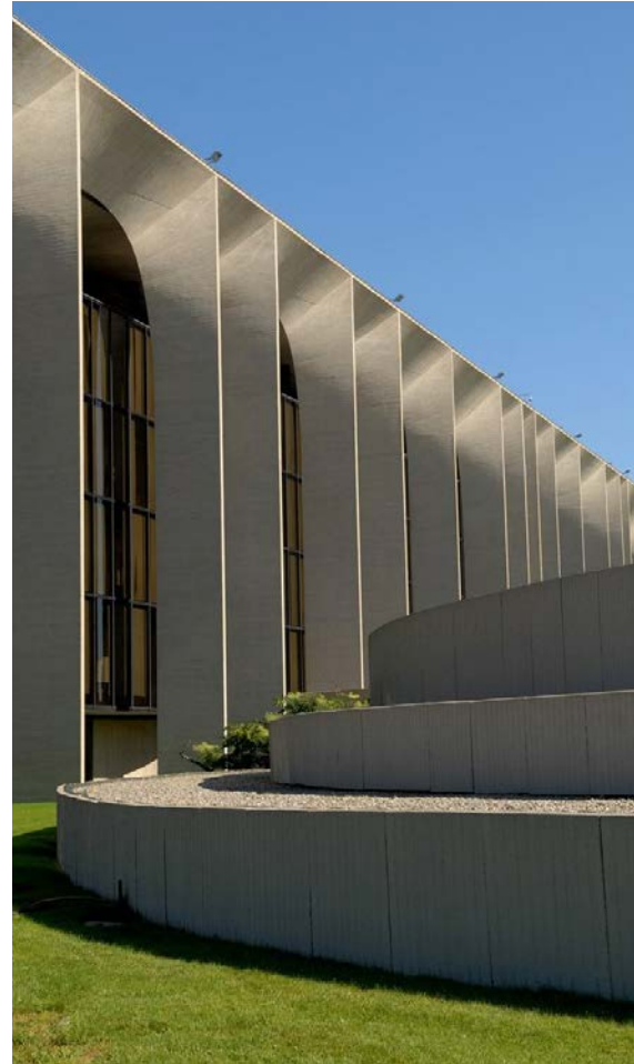
Figure 78: Picture of the columns
