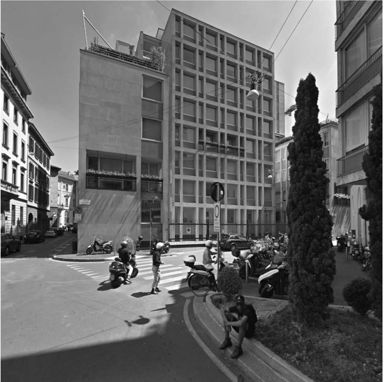
Figure 71: view of building from Piazzatta Bossi
