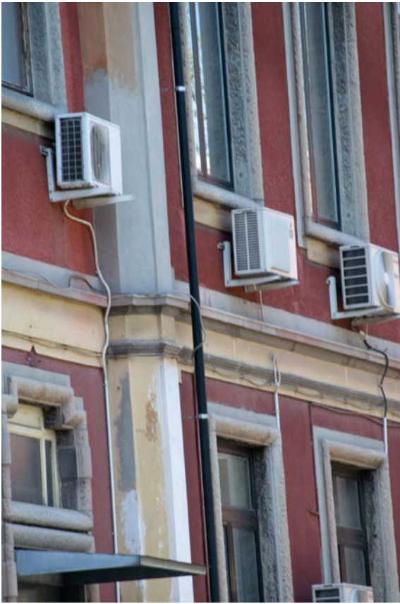
Figure 42: Added elements to the eastern elevation
