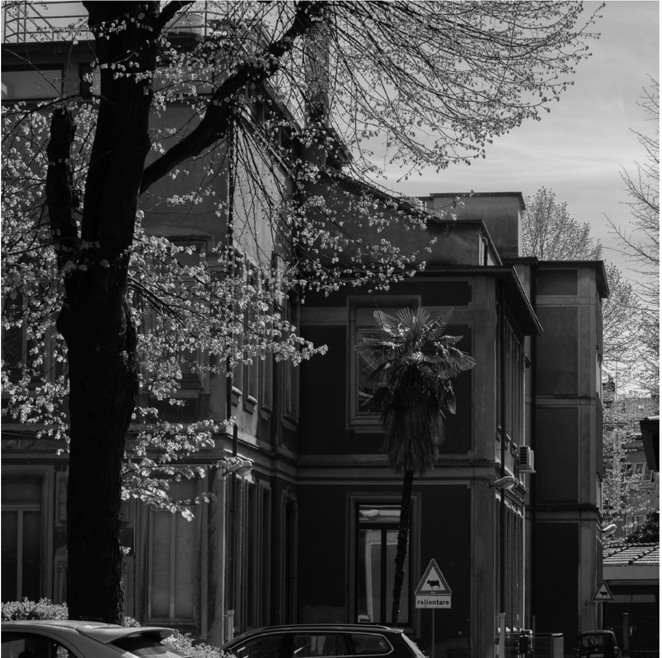
Figure 32: North western view of Building ED22080
