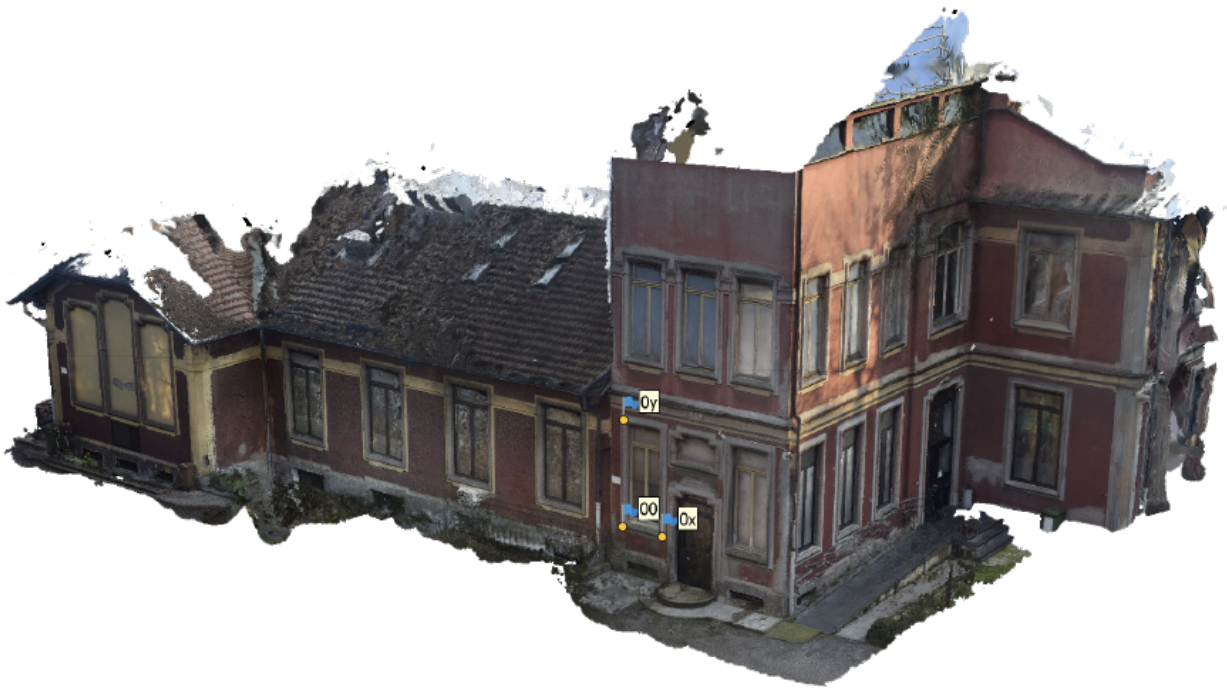
Figure 80: Point Cloud for North-Western elevation
