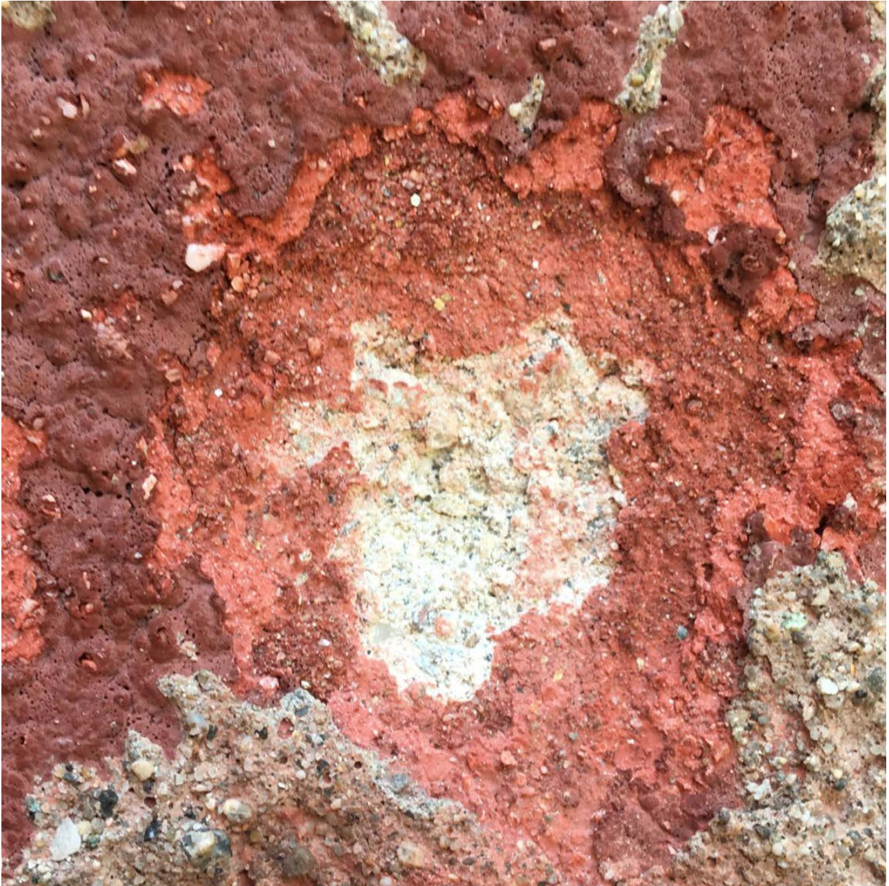
Figure 87: Image of Facade layers of the existing building
