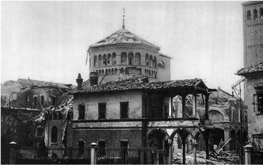
Figure 11: Damage of the Basilica of Sant'Ambrogio
