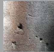
Figure 108: Mechanical damage
