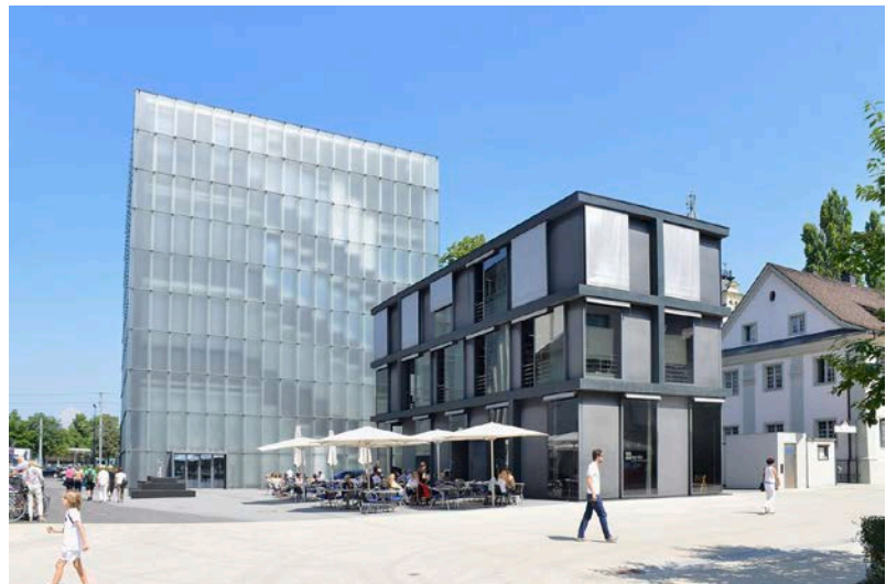
Figure 64: Rear view of building W.r.t to the context
