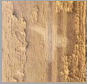
Figure 102: Flacking
