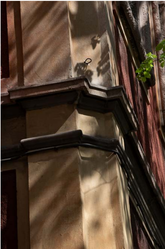
Figure 40: Corner moldings on the existing building
