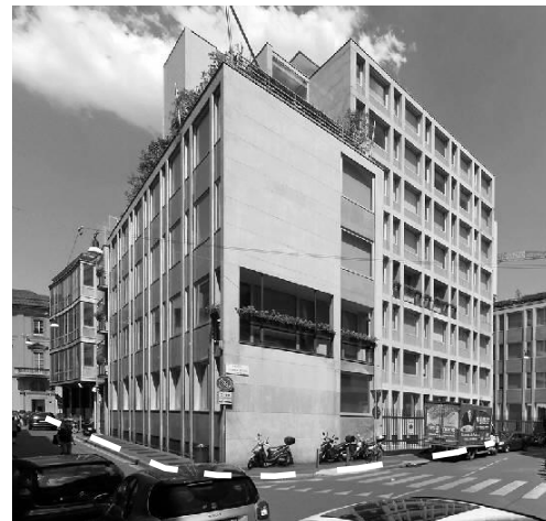
Figure 74: view from north western corner
