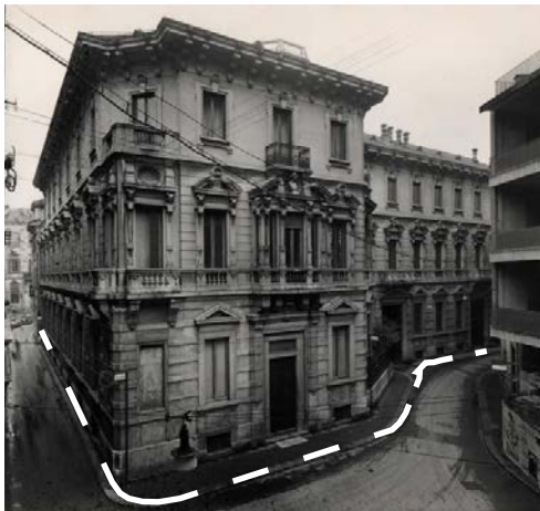
Figure 73: Picture from Piazzata Bossi prior to the construction of the building
