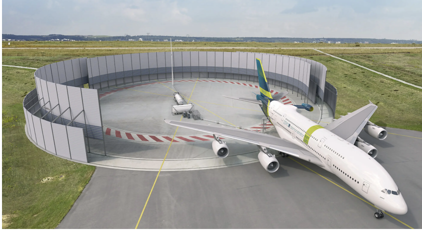
Figure 1.5: Liquid hydrogen refueling station for ZEROe aircraft
