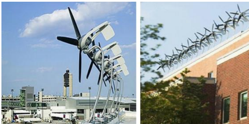
Fig. 2.12 example of retrofitting technology in Boston Logan airport building
