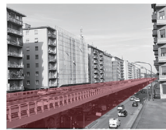
blocking passage lack of bicycle lanes
