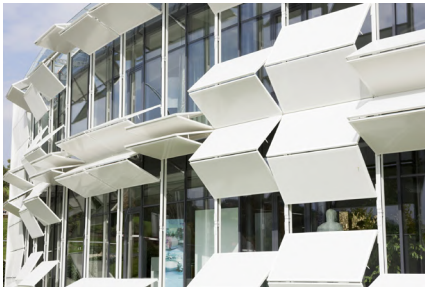
Figura VI.1.26. Kiefer Technic Showroom, Austria
