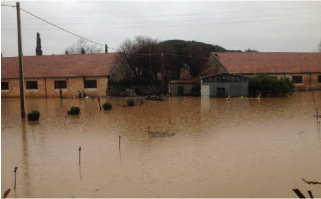
Fig 13. "2014. Flooding of the Centa".
