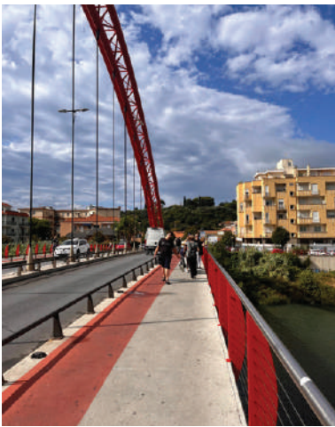
Fig 69. A walk through Ponte rosso [Photography], Note.By Daniela Pico
