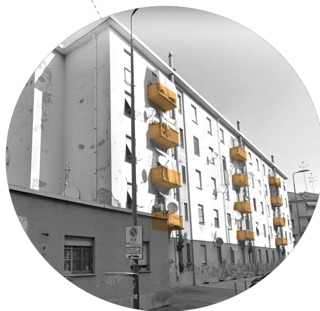
Existing Urban Facade
