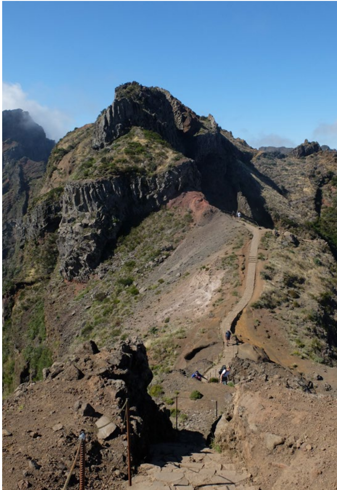
Zone 2 for Proposal C of Siza's Restaurant viewed from the South (ph. L.Pinto)
